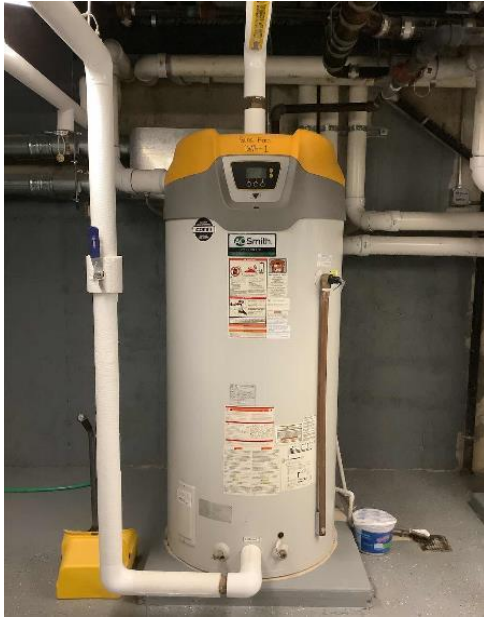
Gas Fired Storage Tank Water Heater
