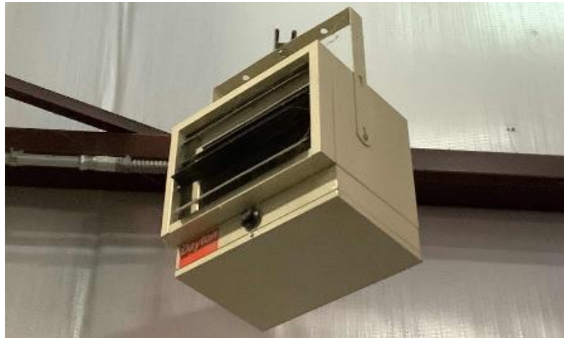
Electric Resistance Heater
