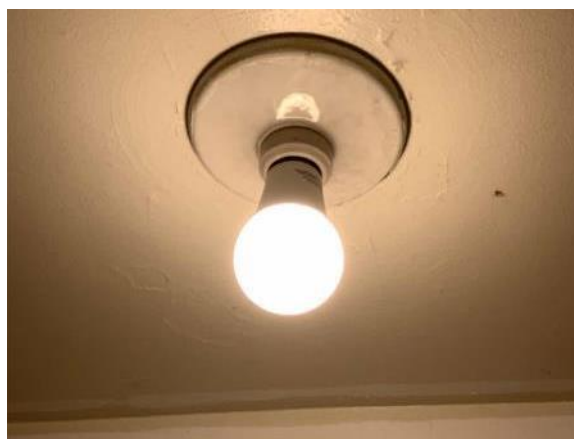
LED Screw-In Lamps
