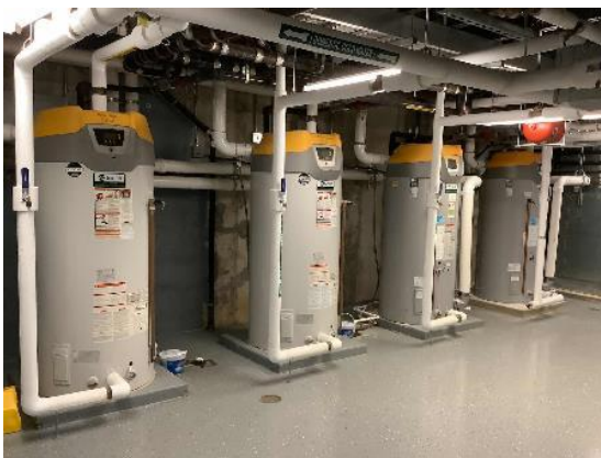
Gas Fired Storage Tank Water Heater
