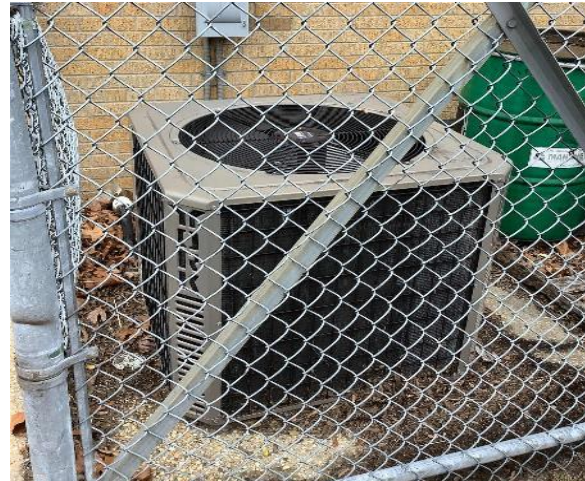
Split AC-Condensing Unit
