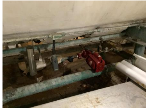
DHW Recirculation Pump
