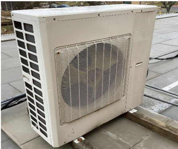
Split AC-Condensing Unit
