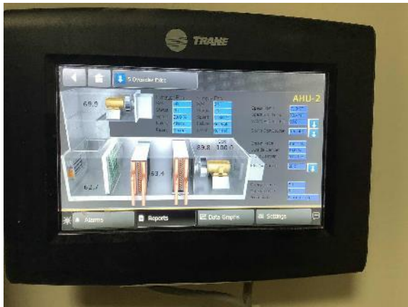
Trane Control System- Air Handling Unit
