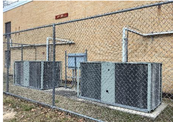
Condensing Unit-Air Handlers
