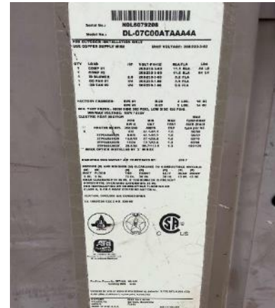
Packaged Rooftop Unit Nameplate
