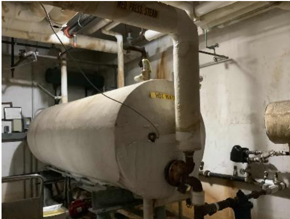
DHW Storage Water Tank
