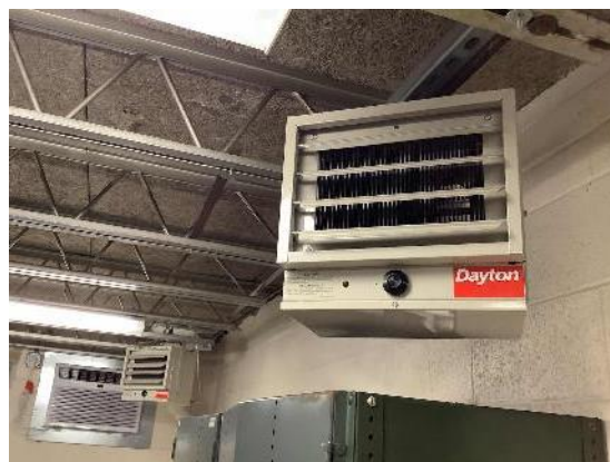
Electric Resistance Heater
