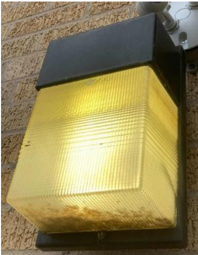
Exterior CFL Wall Pack Fixture
