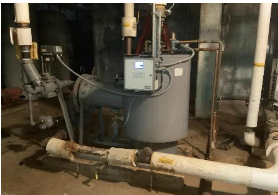
Heat Exchanger-Storage Tank
