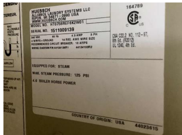
Boiler Nameplate-Laundry System
