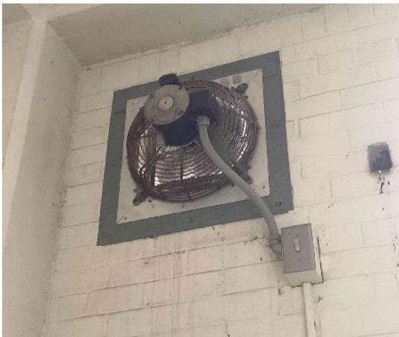
Exhaust Fan-Chemical Room
