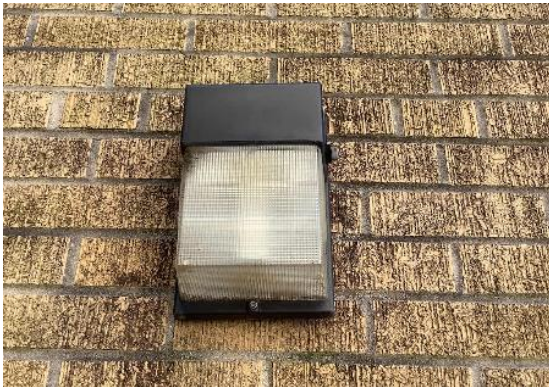
Exterior Oxygen Storage- CFL Wall Pack
