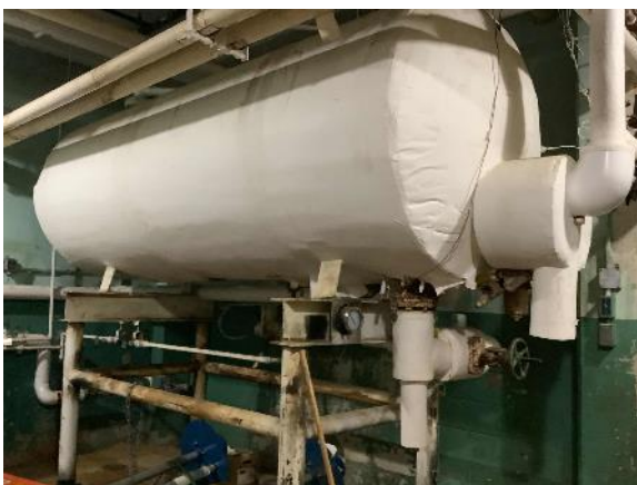
DHW Storage Water Tank
