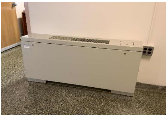
Typical Unit Ventilator
