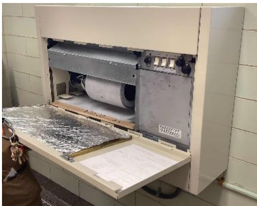
Electric Resistance Unit Heater
