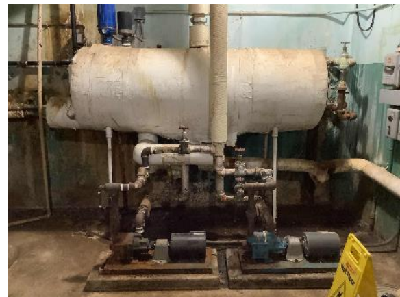
Heating Hot Water Tank- Heat Exchanger
