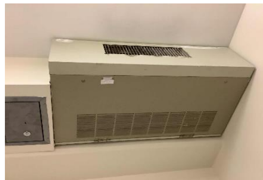
Typical Unit Ventilator
