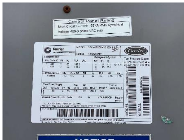
Carrier Chiller Nameplate
