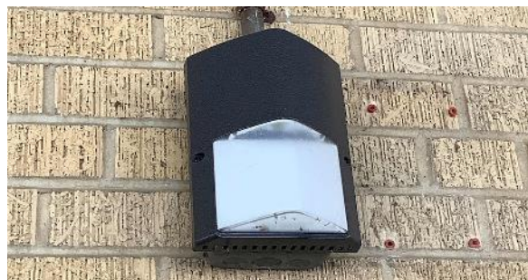
Exterior LED Wall Pack Fixture
