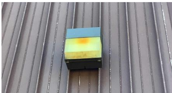
Exterior HID Wall Pack Fixture
