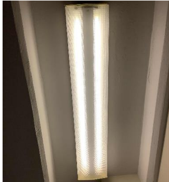
Linear Fluorescent T8 Lamps
