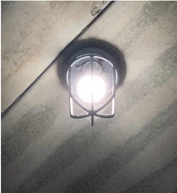
Oxygen Storage – LED Lamps
