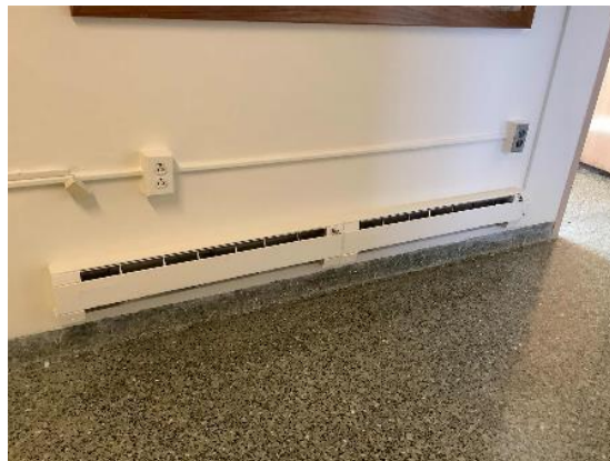
Electric Resistance Unit Heater
