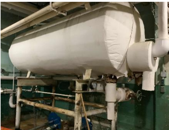
Heating Hot Water Tank- Heat Exchanger
