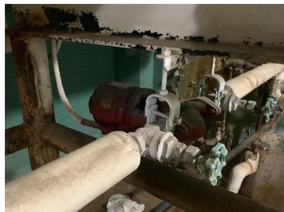
DHW Recirculation Pump
