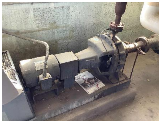
Heating Hot Water Pump
