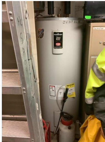
Electric Storage Tank Water Heater
