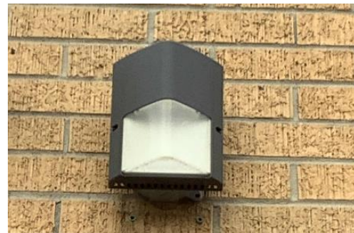
Exterior LED Wall Pack Fixture
