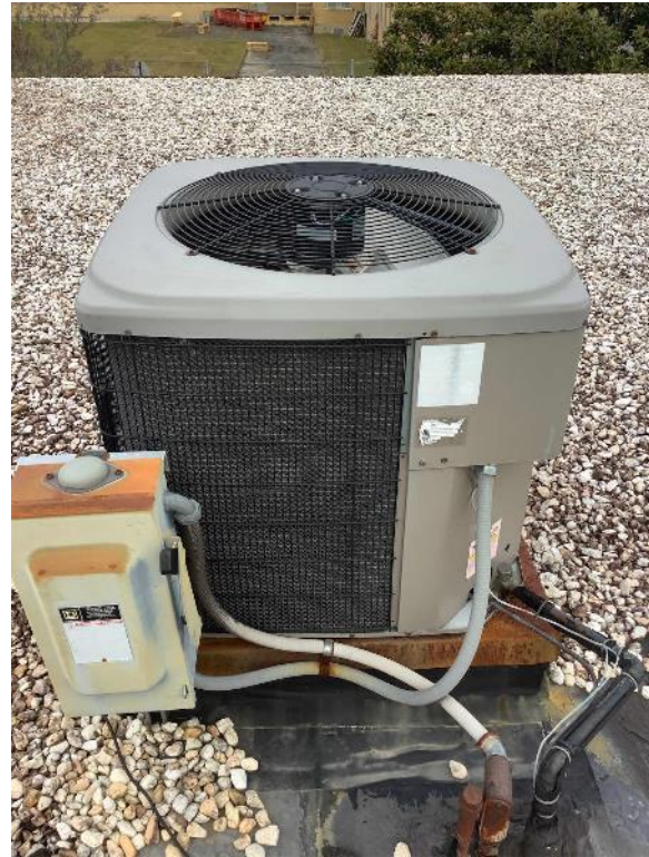
Split AC: Condensing Unit
