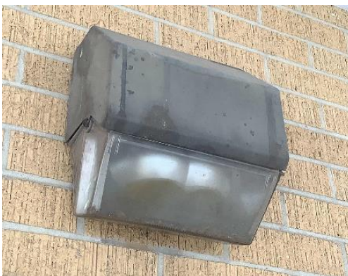
Exterior HID Wall Pack Fixture
