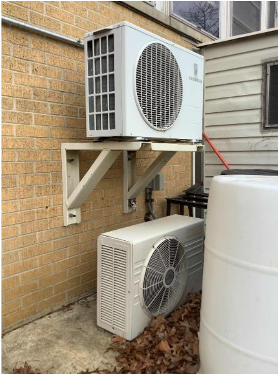
Split AC: Condensing Unit
