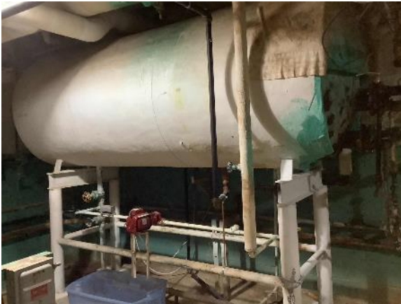
DHW Storage Water Tank
