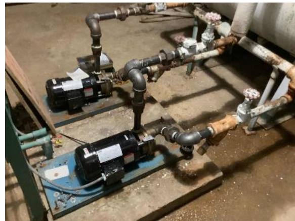
Heating Hot Water Pumps
