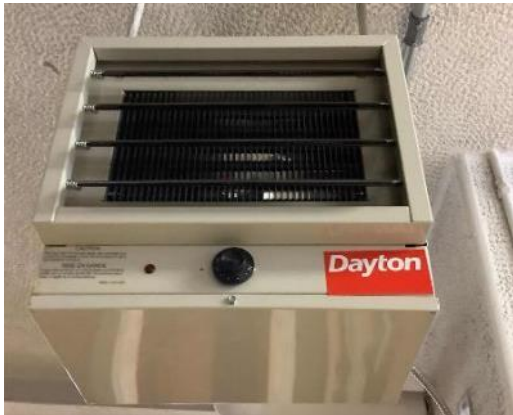
Electric Resistance Heater
