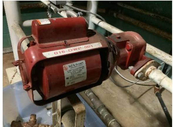
DHW Recirculation Pump
