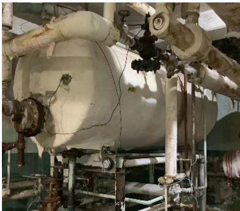
DHW Storage Water Tank
