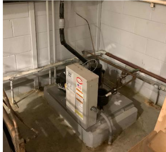
Air Cooled Condenser-Refrigeration
