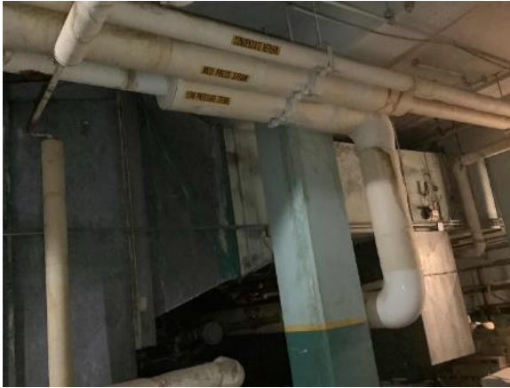
Steam Piping-Air Handling Unit
