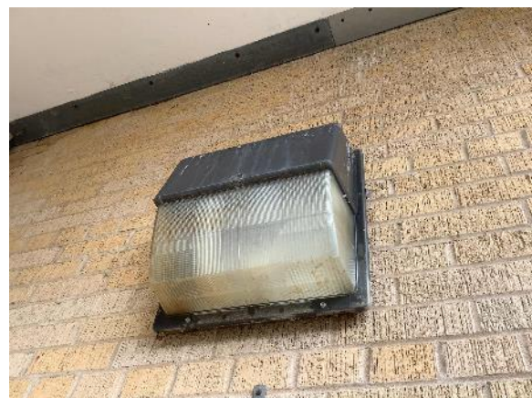
Exterior HID Wall Pack Fixture
