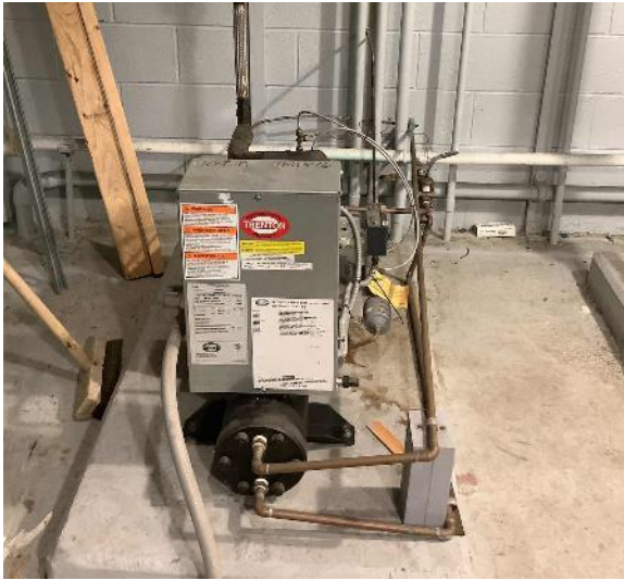
Water Cooled Condenser-Refrigeration
