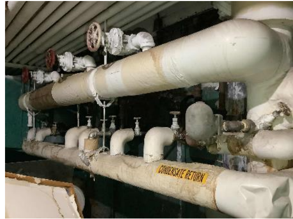
Steam Piping-Air Handling Unit
