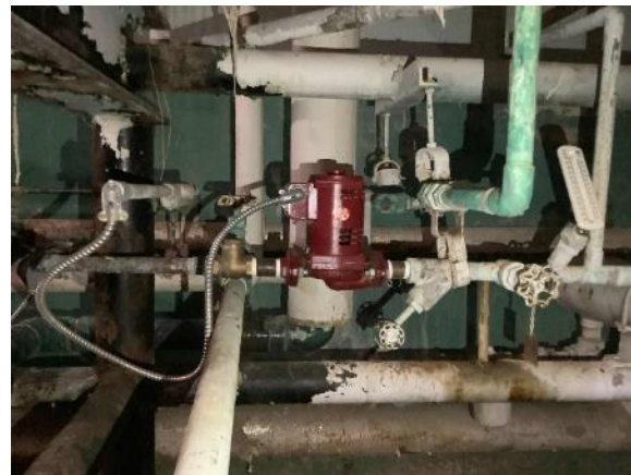
DHW Recirculation Pump
