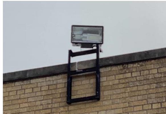
Exterior LED Fixture
