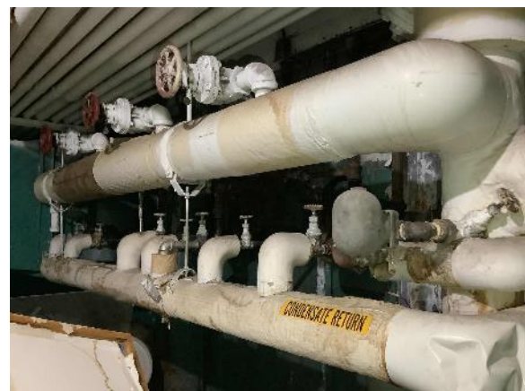
Air Handling Unit- team Piping
