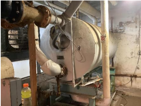
Heat Exchanger- Storage Tank
