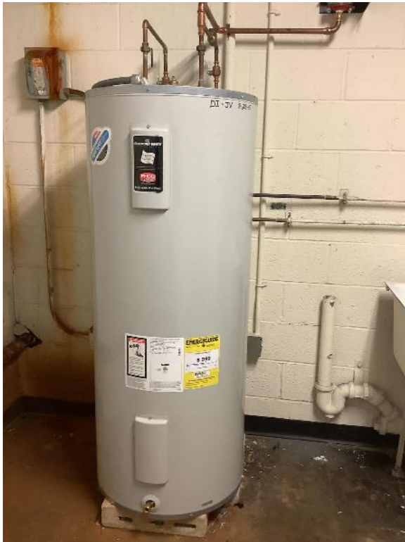
Electric Storage Tank Water Heater
