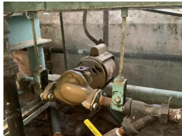
Heating Hot Water Pump
