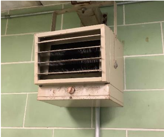
Electric Resistance Heater: Chlorine Building
