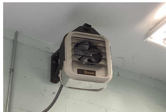
Electric Resistance Heater: Lift Station
