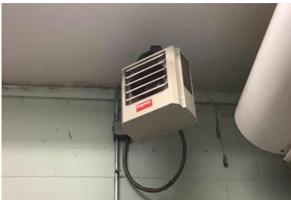
Electric Resistance Heater: Lift Station
