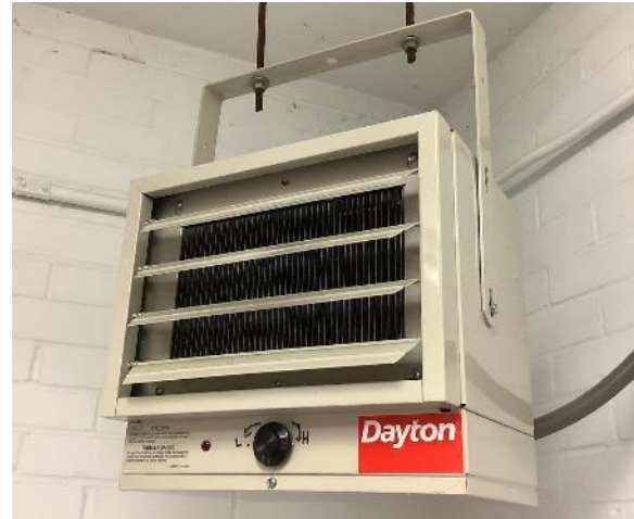
Electric Resistance Heater: Office Building
