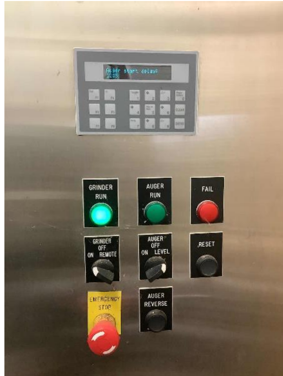
Control Panel: Lift Station
