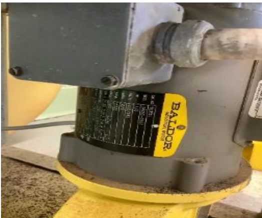
Chlorine Mixing Motors
