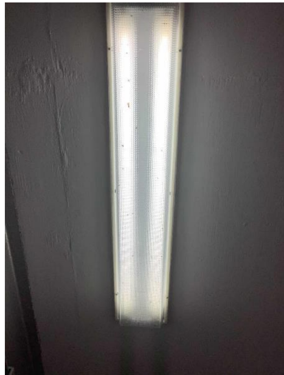
Typical T8 Linear Fluorescent Lamps
