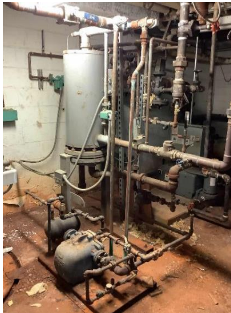
Hot Water Tank–Heat Exchanger–Spruce Hall
