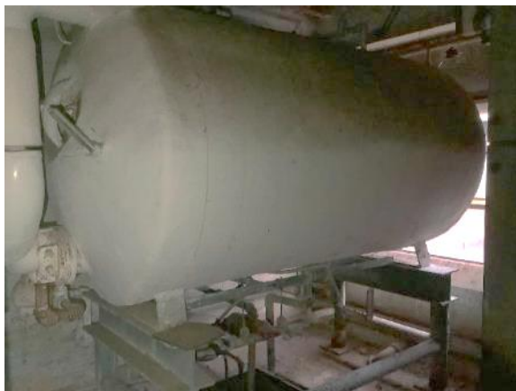
Heating Hot Water Tank-Hemlock Hall
