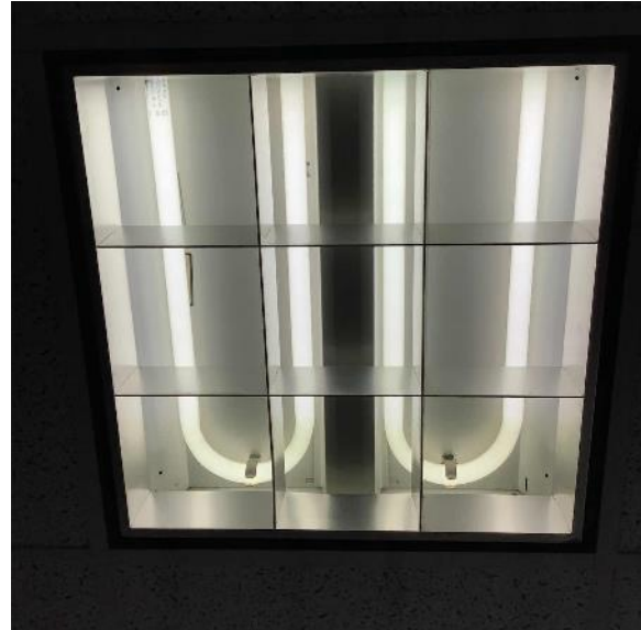
Linear Fluorescent U-Bend T8 Lamps-Spruce Hall
