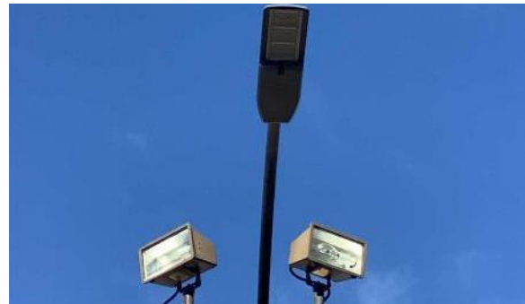
Pole Fixture-HID and LED Fixture (Mix)-Hemlock Hall
