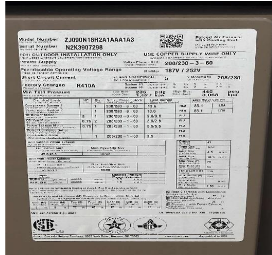
New Carrier RTU with Natural Gas-Fired Heater Installed in February 2024
