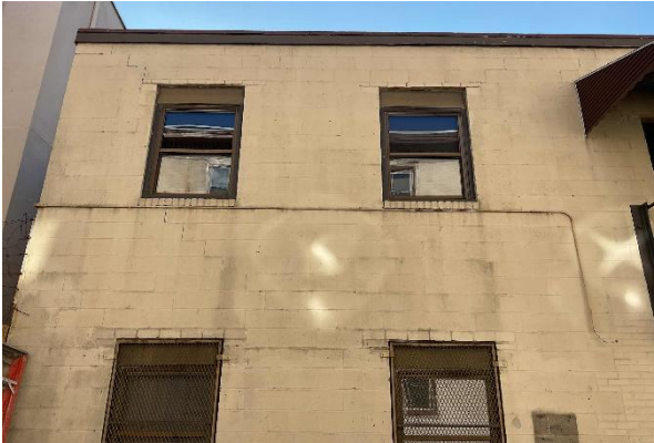
Typical Double Pane Glass Windows with Aluminum Frames
