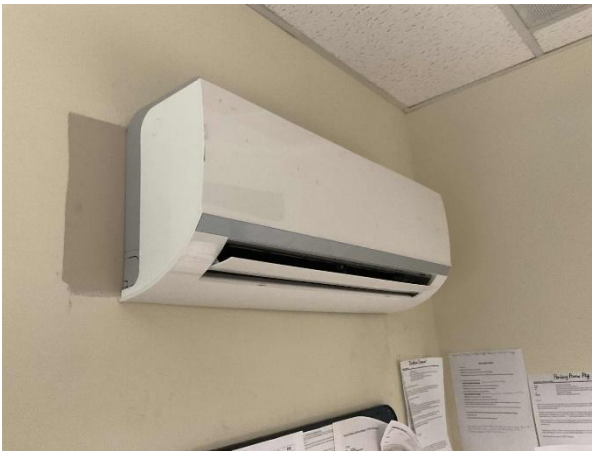
Carrier Split-System Air Conditioner Unit
