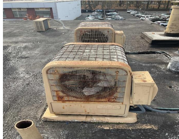
Left: Electric Resistance Heater in Elevator Room & Right: York Condensing Units Attached to Borg-Warner Furnaces
