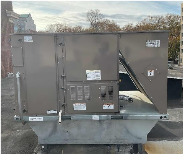
New Carrier RTU with Natural Gas-Fired Heater Installed in February 2024
