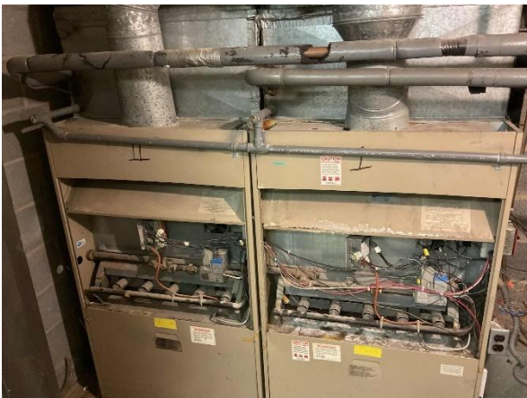
Borg-Warner Natural Gas Furnaces Installed in 1984
