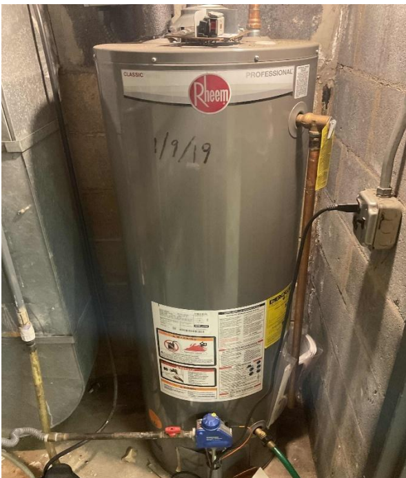
Rheem Natural Gas Storage Tank Water Heater
