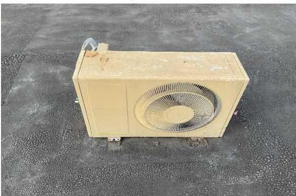
Dynazone Split-System Air Conditioner Unit
