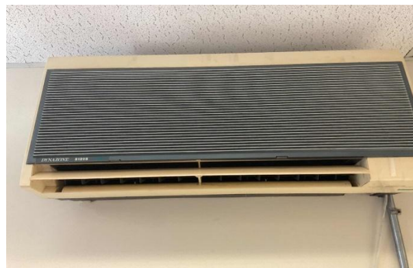
Dynazone Split-System Air Conditioner Unit
