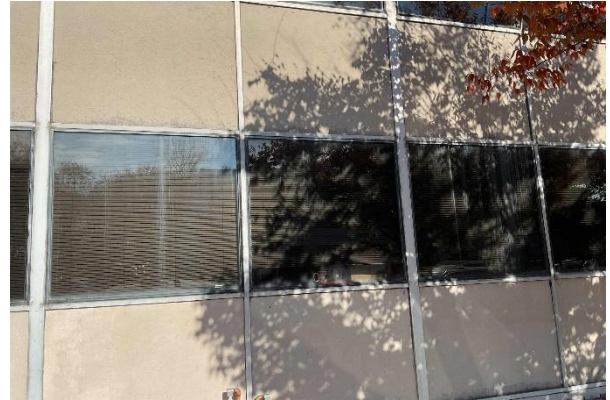
Typical Double Pane Glass Windows with Aluminum Frames
