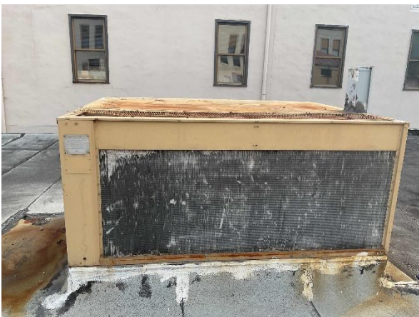
Borg-Warner Cooling-Only RTU Installed in 1984
