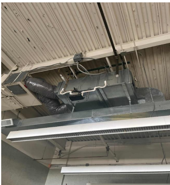
Fireman's Storage Air Handling Unit
