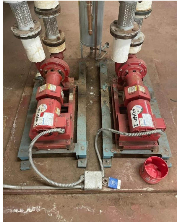
Heating Hot Water Pumps
