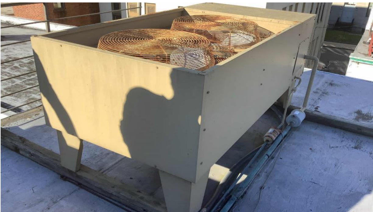
Split System AC Condenser
