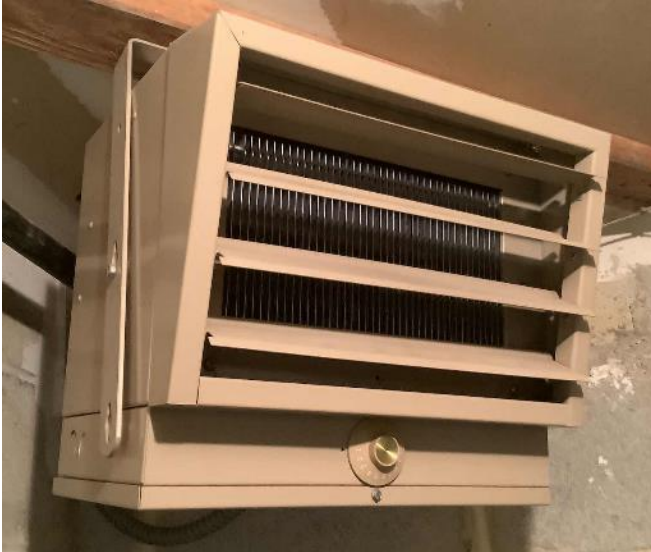
Electric Resistance Heaters
