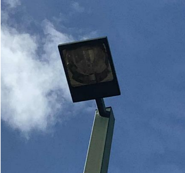
Exterior MV Fixture
