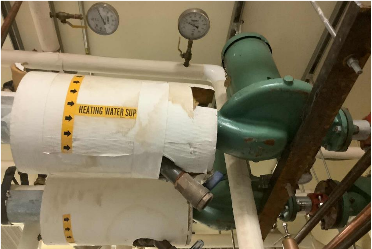
Heating Hot Water Pumps
