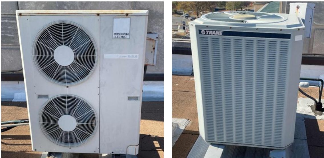
Split System Air Source Heat Pump & AC Condensing Unit
