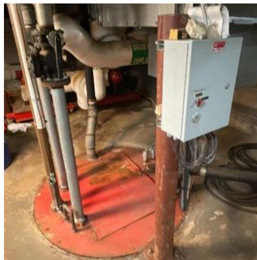
Sewer Ejector Pump
