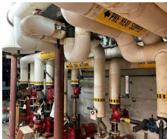
HHW Pumps & Insulated Pipes
