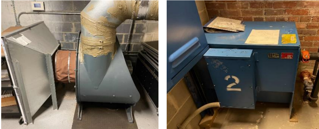
Pipe Organ Air Supply Motor & Elevator Motor
