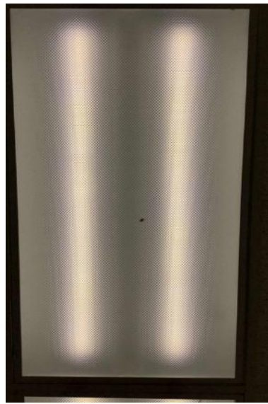
4-Foot T8 Equivalent LED Linear Tubes
