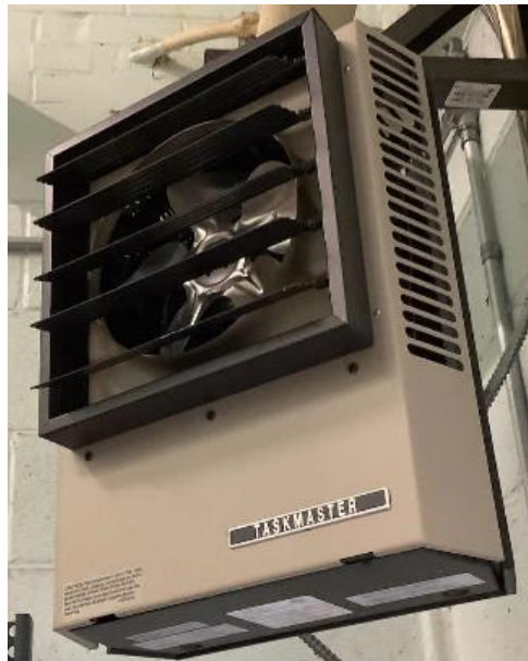
Sprinkler Room Electric Resistance Heater
