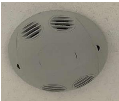
Ceiling Mounted Occupancy Sensor
