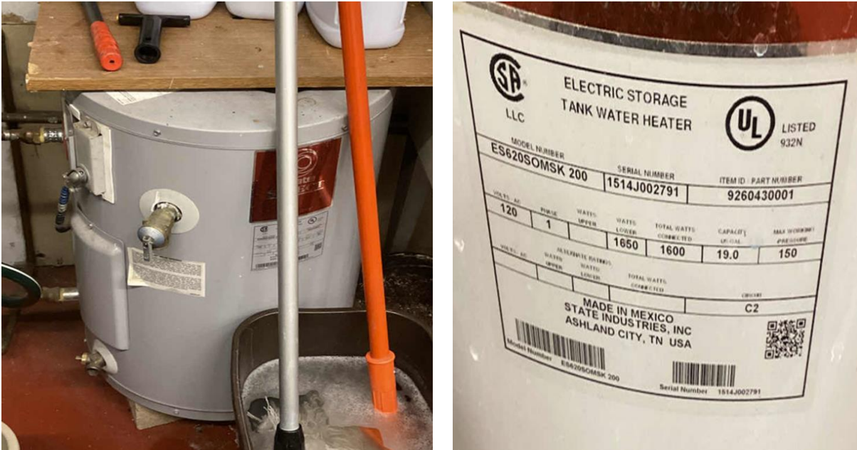
First Floor Electric Domestic Hot Water Heater
