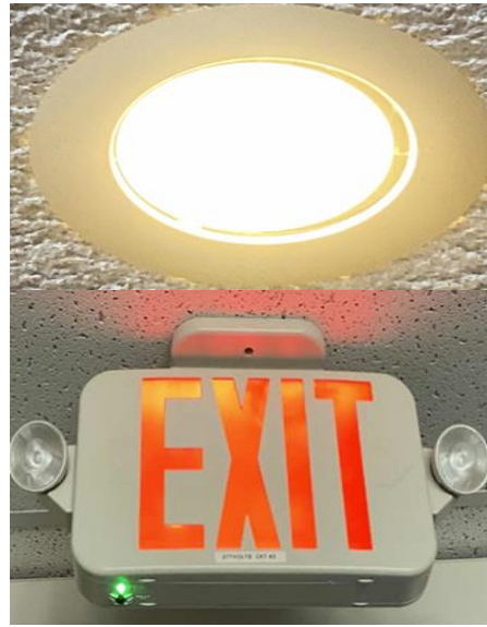
2 Foot LED Fixture, CFL Recessed Can & LED Exit Sign
