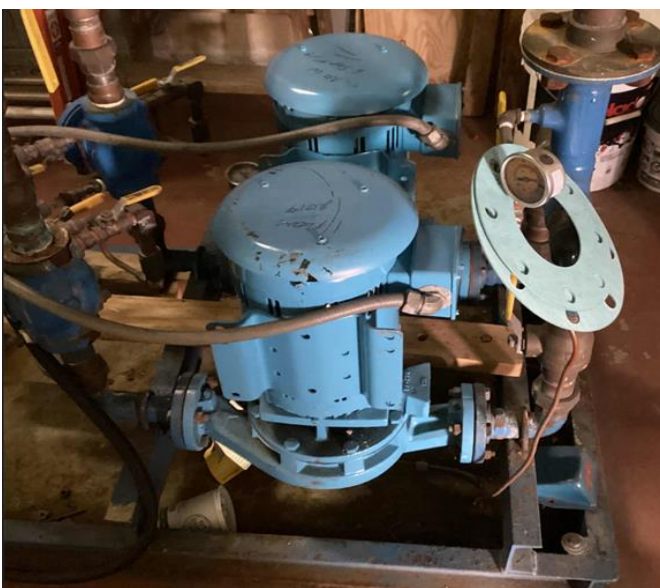
7.5 hp Heating Hot Water Pumps
