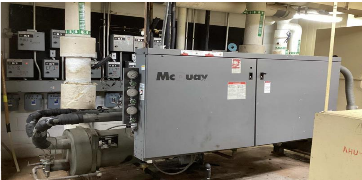
Water-Cooled Reciprocating Chiller
