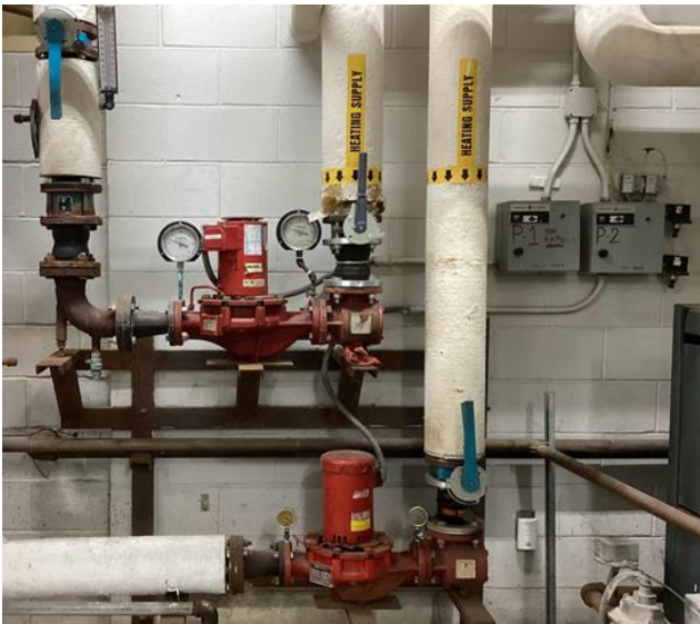
Heating Hot Water Pumps
