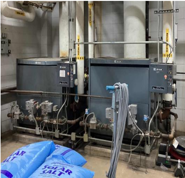
Heating Hot Water Boilers
