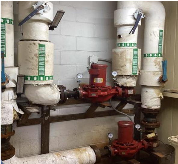
Chilled Water Pumps & Tag
