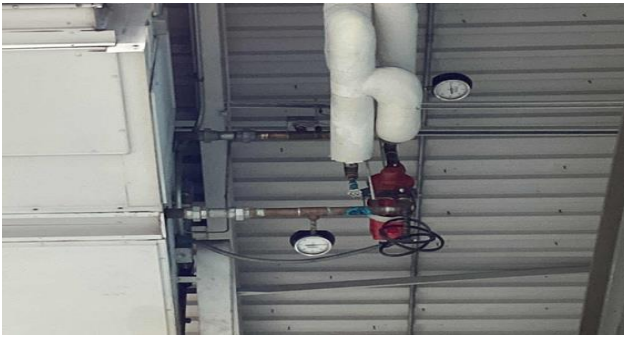
Unit Vent Heating Hot Water Pumps
