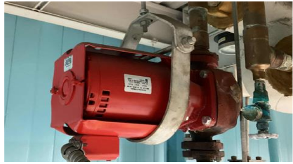
Unit Vent Heating Hot Water Pumps
