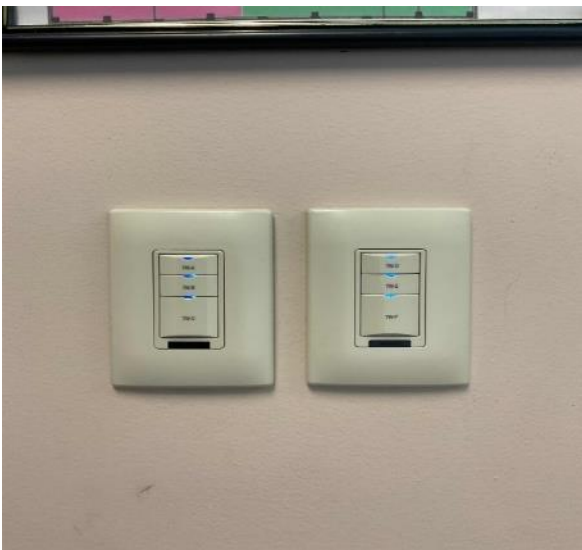
Left: Wall Switches Connected to Watt Stopper Automation System, Right: Typical Occupancy Sensor
