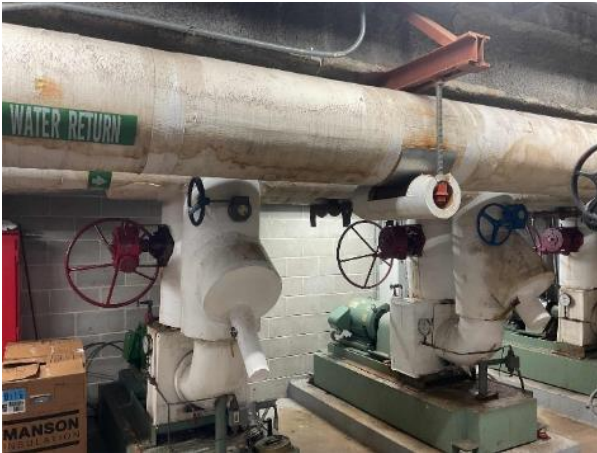
Chilled Water Pipes with Insulation
