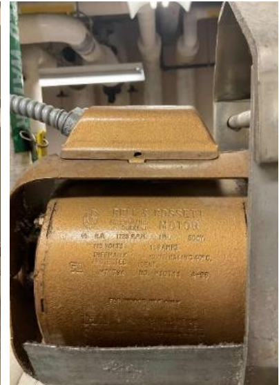
Typical Domestic Hot Water Circulation Pump
