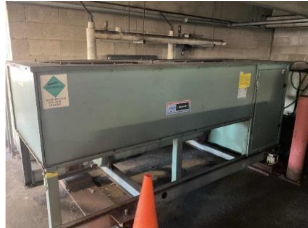
Garage Chiller Condensing Unit
