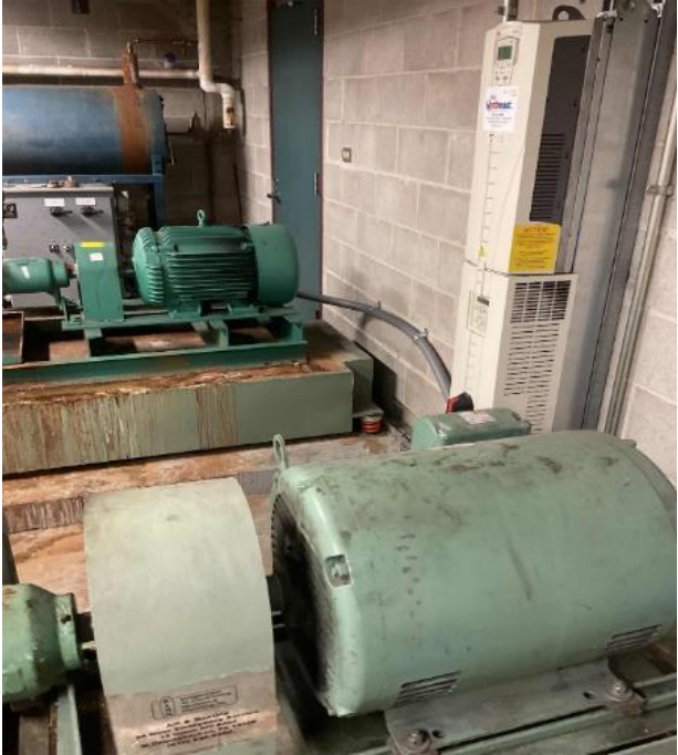
Typical Heating Hot Water Pump Motors
