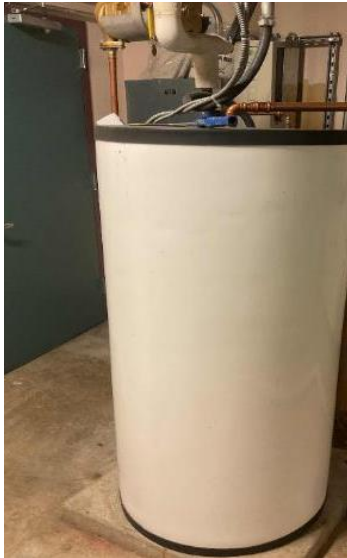
Typical Storage Tank Electric Water Heater
