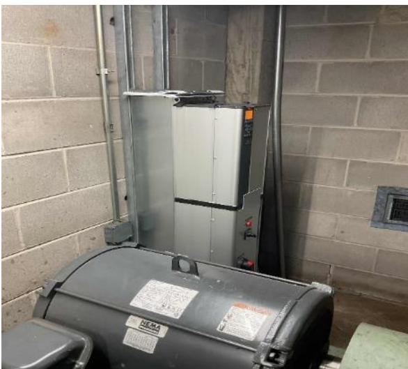
Typical Chilled Water Pump Motor with Attached VFD
