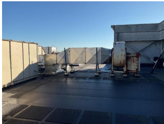
Main Building Roof with Black Rubber Membrane
