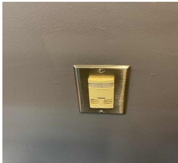
Left: Wall Switches Connected to Watt Stopper Automation System, Right: Typical Occupancy Sensor
