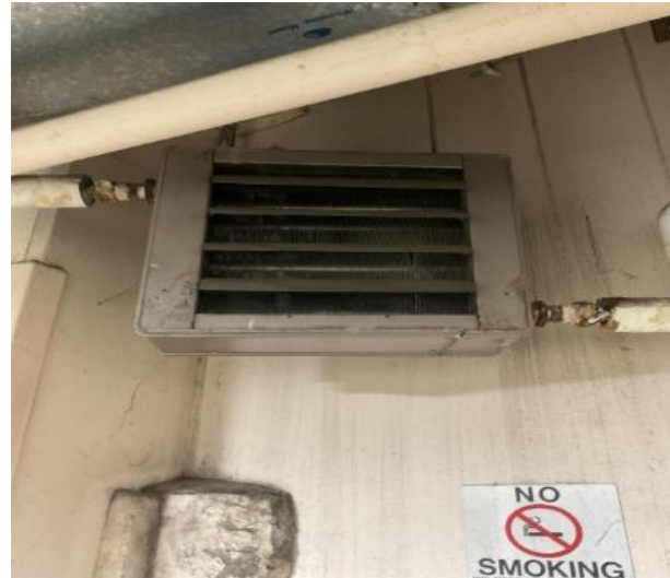
Typical Hot Water Unit Heaters
