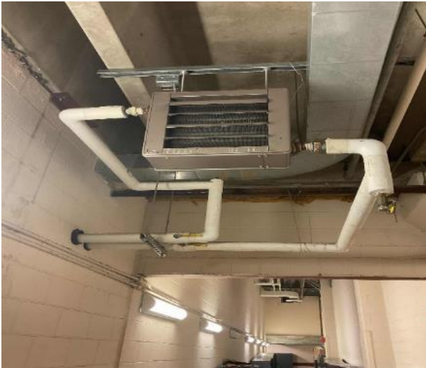
Typical Hot Water Unit Heaters
