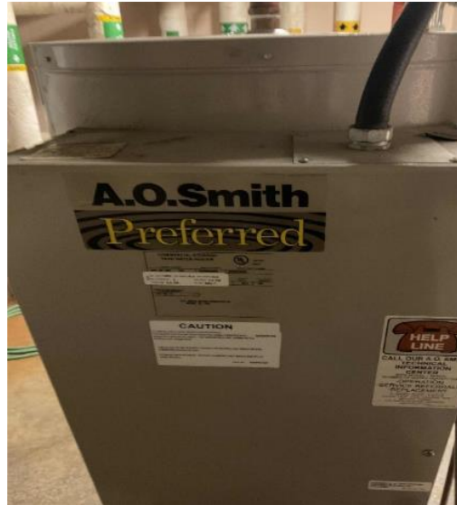
Typical Storage Tank Electric Water Heater
