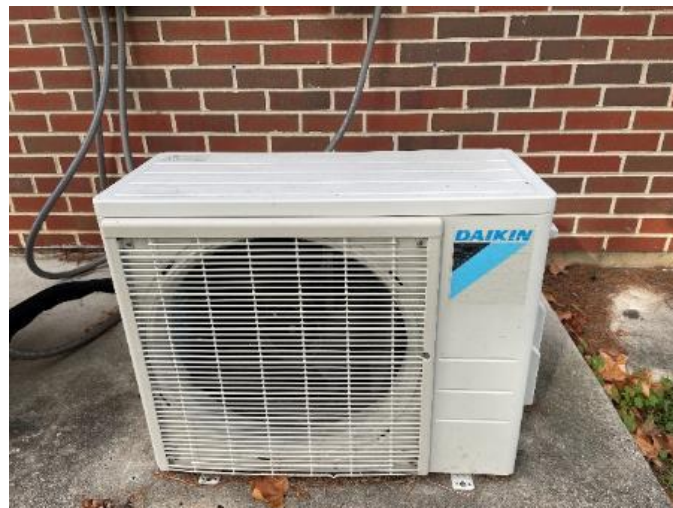
Ductless Mini-Split Unit
