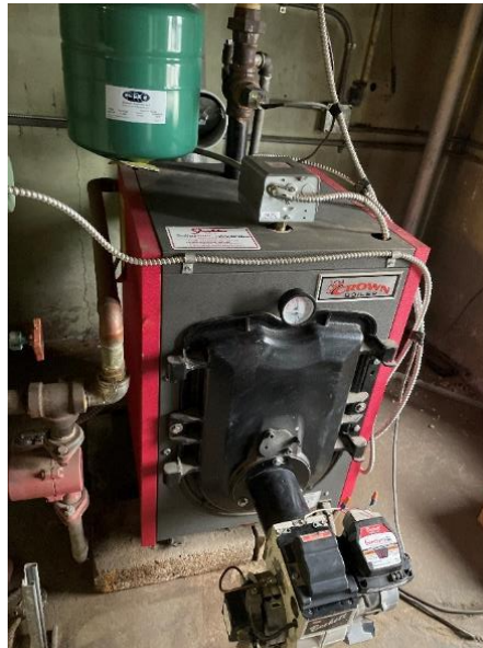
Hydronic Boiler (Paint Shop)
