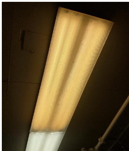
Linear Fluorescent T8 Fixture
