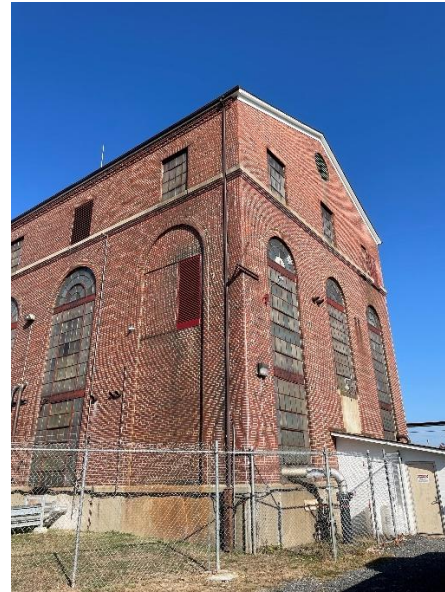
Side of Building
