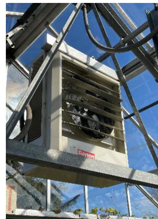
Greenhouse #2 Unit Heater-Electric
