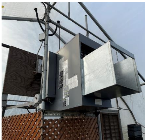
Greenhouse #1 Unit Heater-Propane
