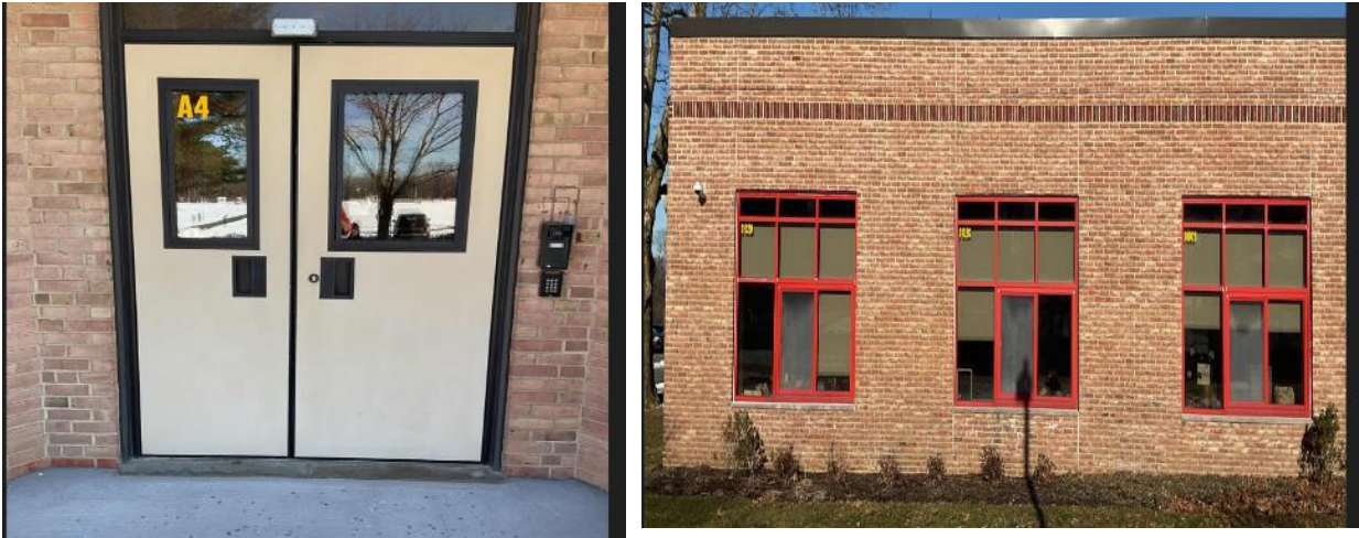
Exit Door & Typical Window
