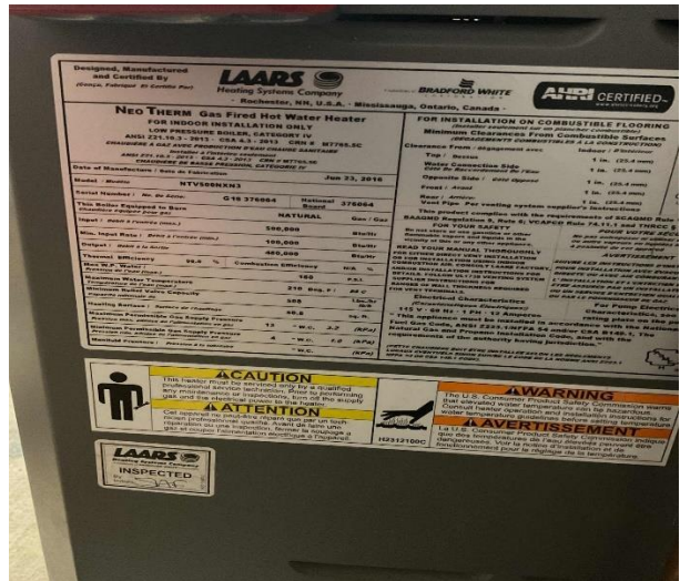
Domestic Hot Water Boiler
