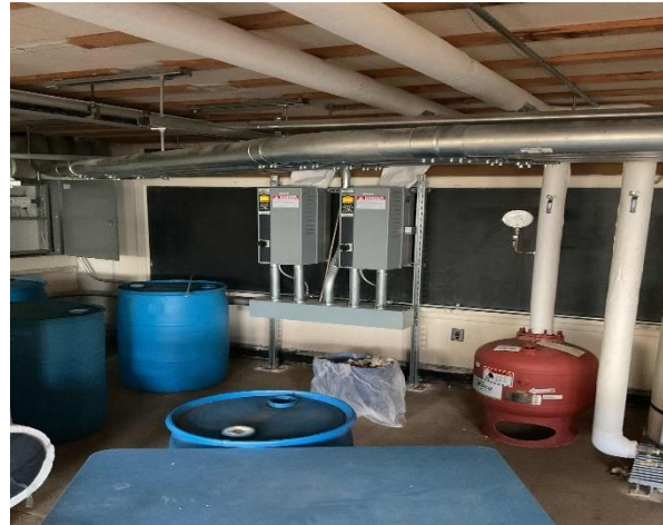
Chilled Water Pumps with Attached VFDs
