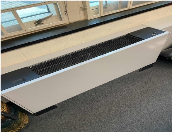
Typical Unit Ventilators
