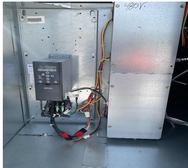
Typical ECM Supply Fan Motor & Attached VFD
