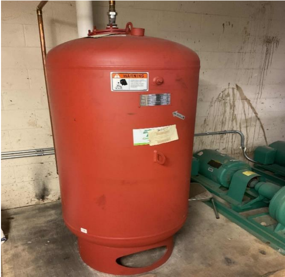
Domestic Hot Water Storage Tank
