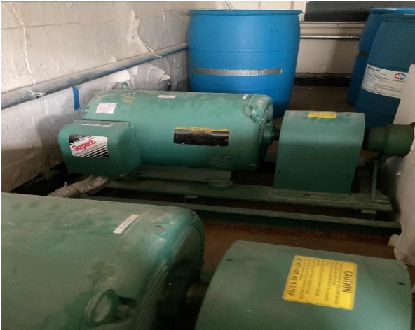
Chilled Water Pumps with Attached VFDs
