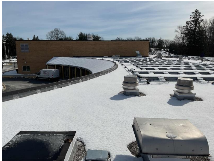
Facility Rooftop & Solar Array
