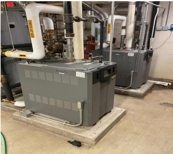
Domestic Hot Water Boiler
