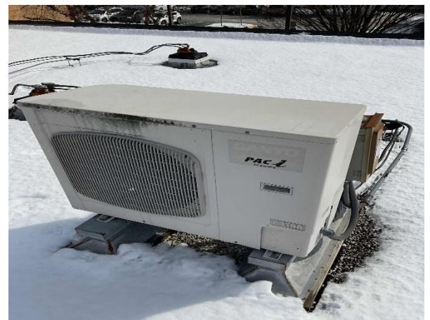
Typical Split System Units
