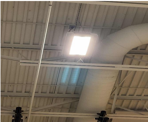
Gymnasium LED High Bay Lighting & LED Light Panels
