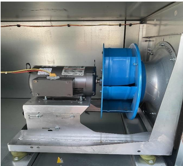
Typical ECM Supply Fan Motor & Attached VFD
