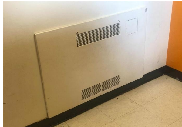
Unit Ventilator and Fan Coil Unit
