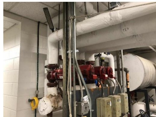
Hot Water Boilers and Heating Hot Water Pumps
