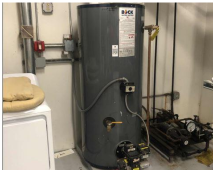
Oil Fired Hot Water Heater and DHW Pumps
