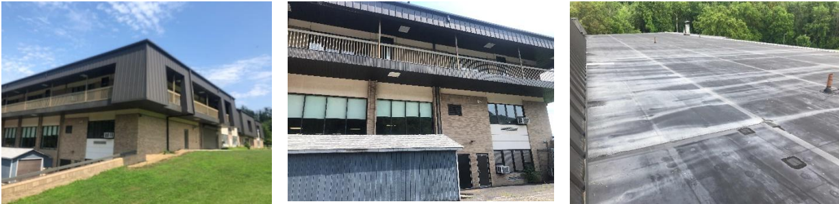
Building Exterior and Roof
