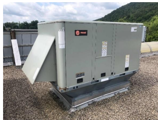
PTHP and Packaged RTU
