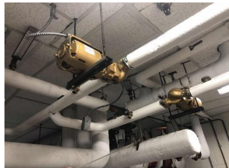
Oil Fired Hot Water Heater and DHW Pumps
