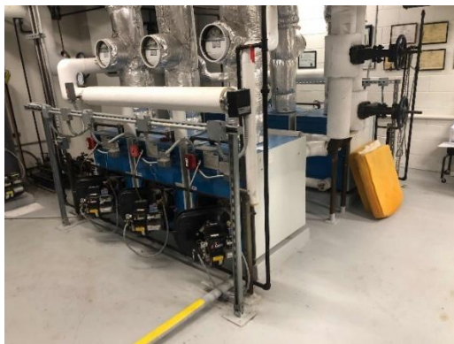
Hot Water Boilers and Heating Hot Water Pumps
