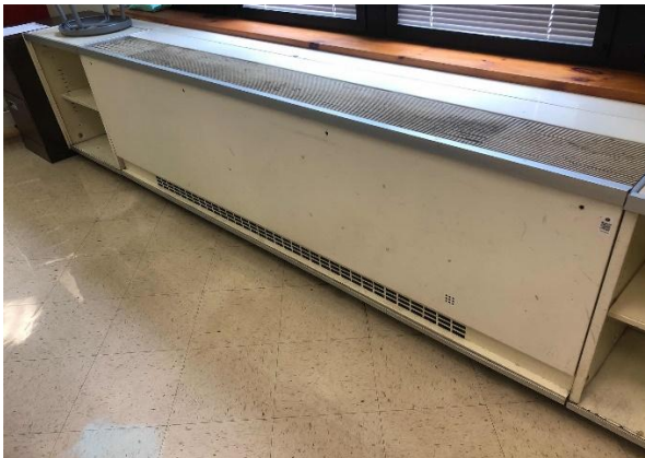
Unit Ventilator and Fan Coil Unit
