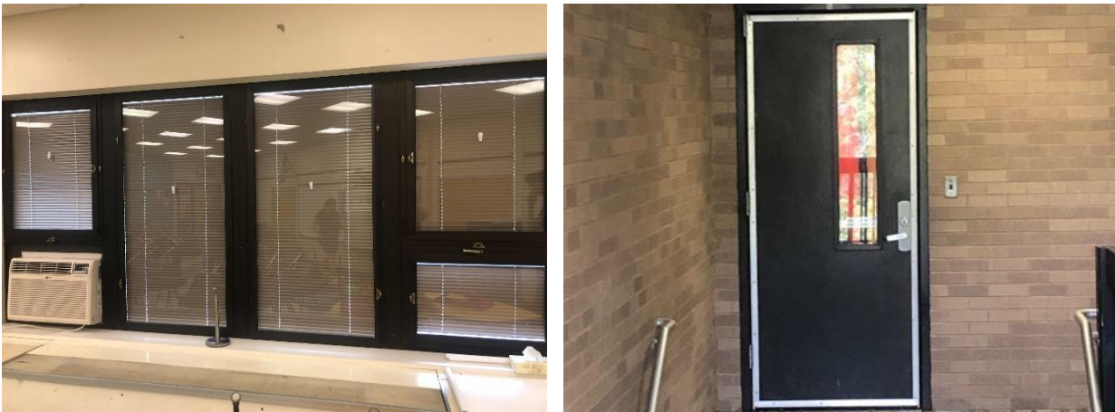
Windows and Exterior Door
