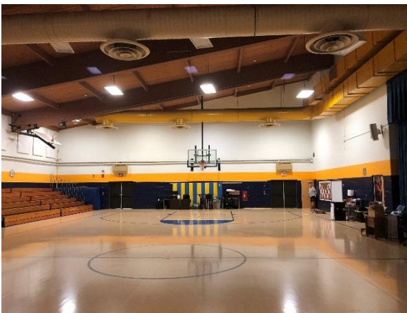
Linear Fluorescent and LED fixtures
