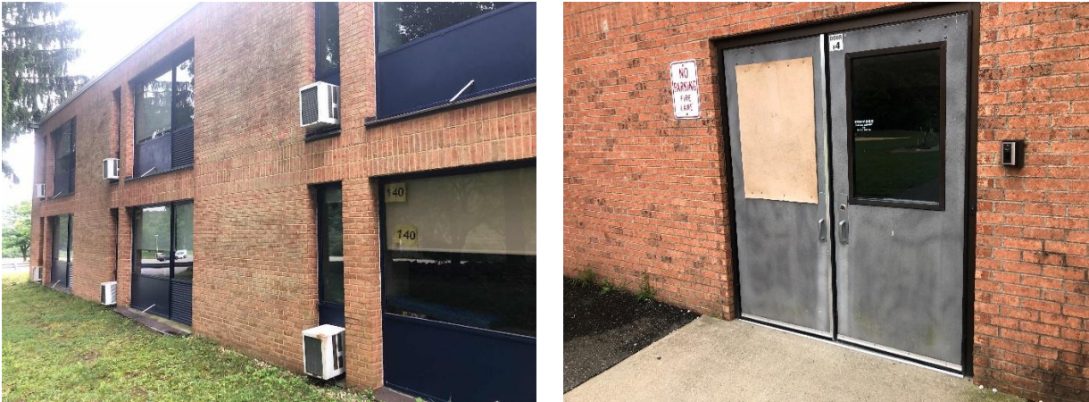
Windows and Exterior Door
