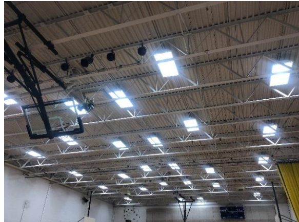
Linear Recessed Troffer and Surface Mounted Fixtures
