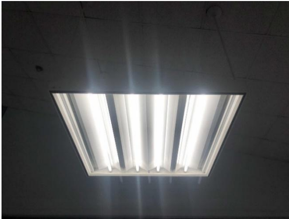
Linear Recessed Troffer and Surface Mounted Fixtures
