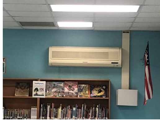
Mini Split System Outdoor Unit and Indoor Console.
