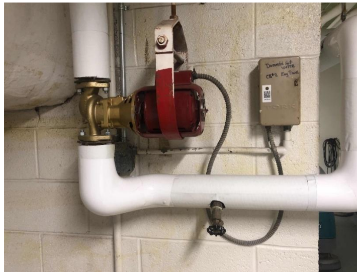
Storage Tank Water Heater and Circulation Pump
