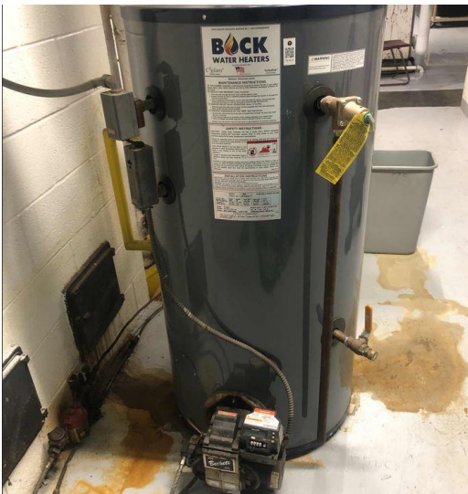
Storage Tank Water Heater and Circulation Pump
