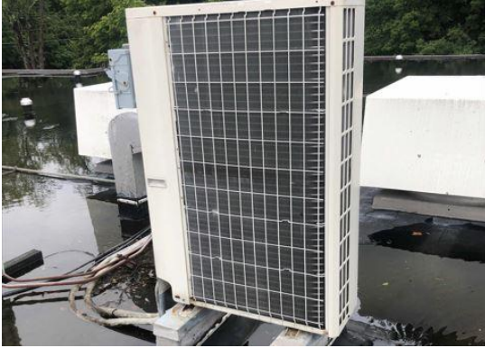
Mini Split System Outdoor Unit and Indoor Console.
