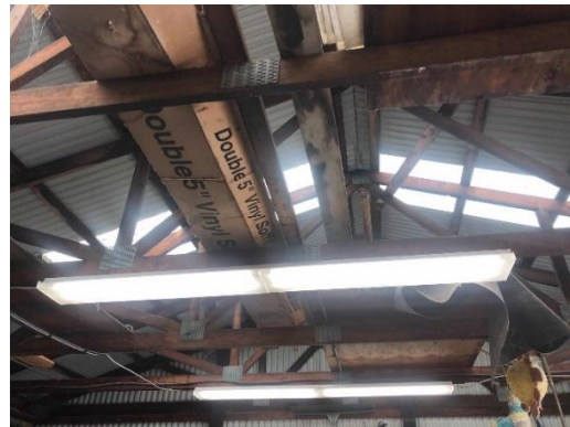
Linear LED and Fluorescent Fixtures
