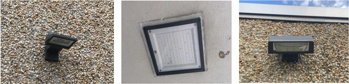
LED Wall Packs, Canopy, and Flood Light Fixtures
