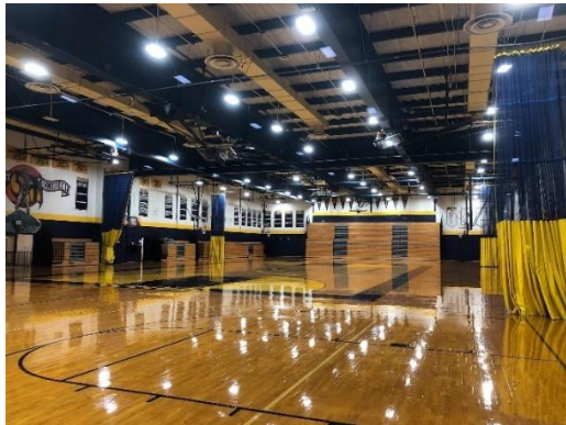
Linear LED and Fluorescent Fixtures
