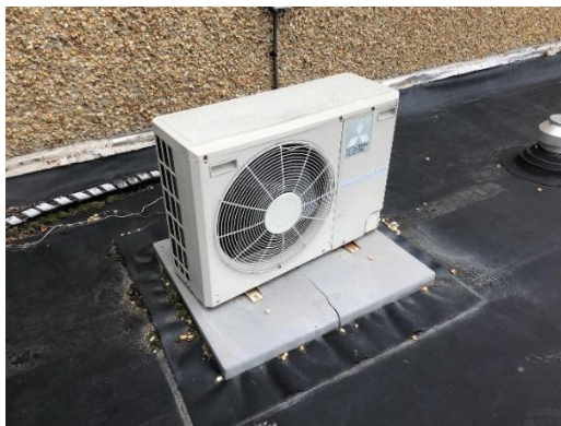
Outside Condensing Unit and Indoor Unit
