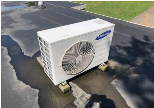
Outside Condensing Unit and Indoor Console
