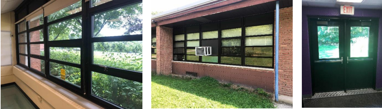
Windows and Exterior Door
