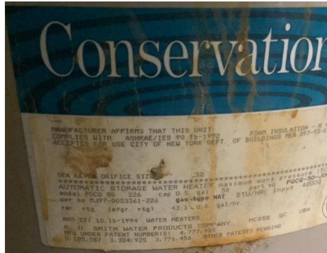
Hot water heater nameplate
