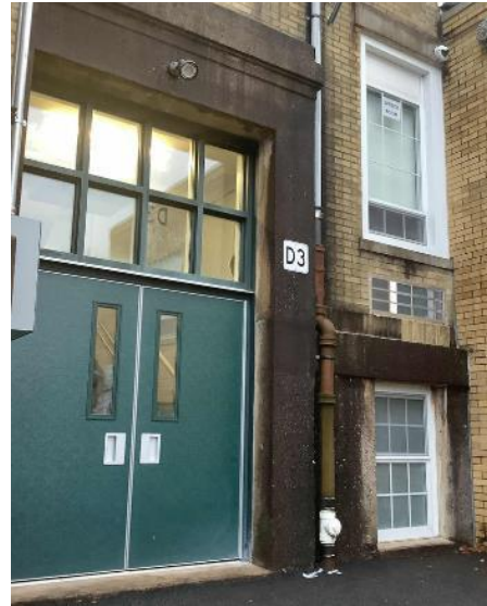
Windows and door
