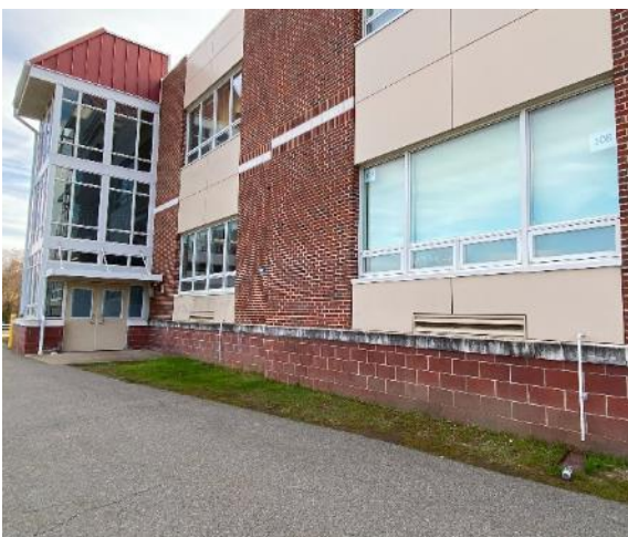
Rear Stair Well
