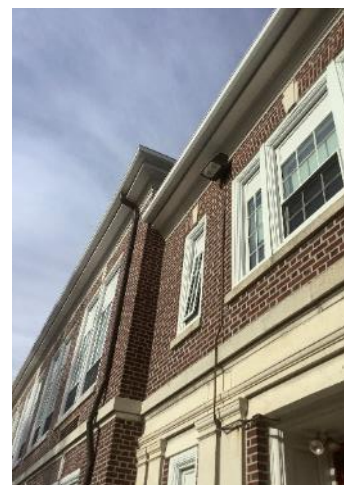
Windows on Original Building Section
