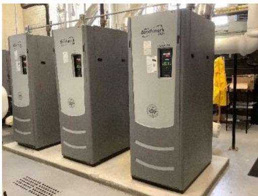
Condensing Boilers
