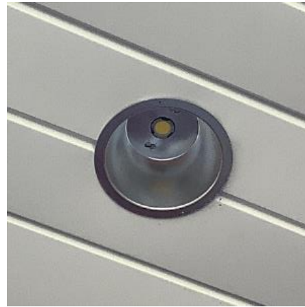
Recessed Can LED hardwire fixture
