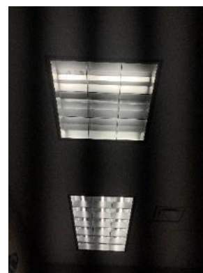
Recessed Parabolic
