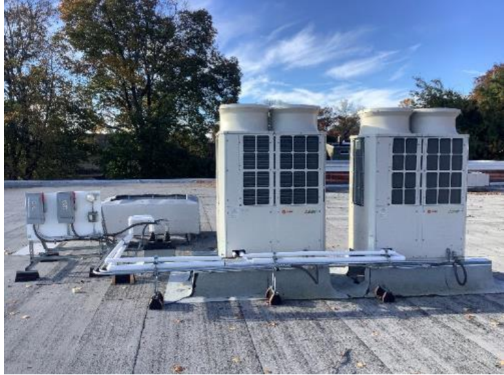
VRF Split System Heat Pumps
