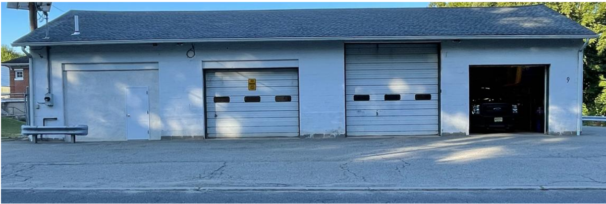
Garage Doors and Building Facade
