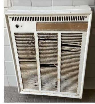
Electric Resistance Heater
