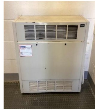
Electric Resistance Heater
