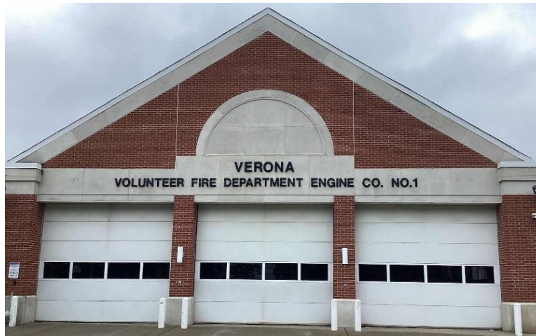
Firehouse Garage Doors
