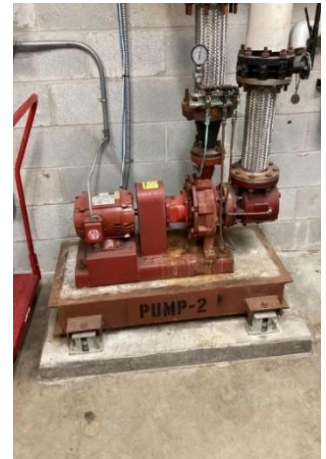
Heating Hot Water Pumps
