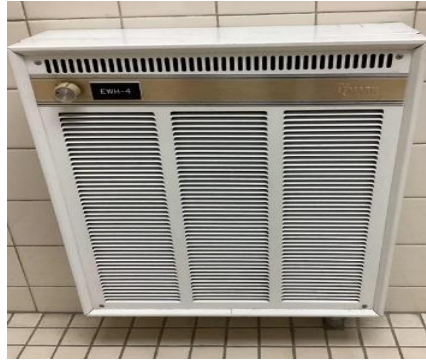
Electric Resistance Heater
