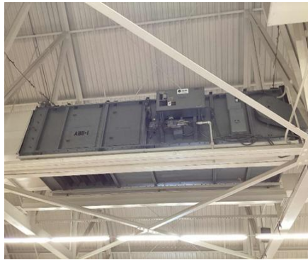
AHU-1 Furnace
