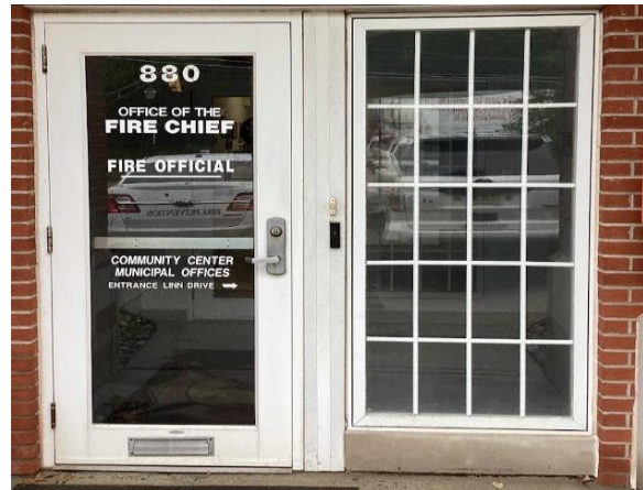
Community Center Door
