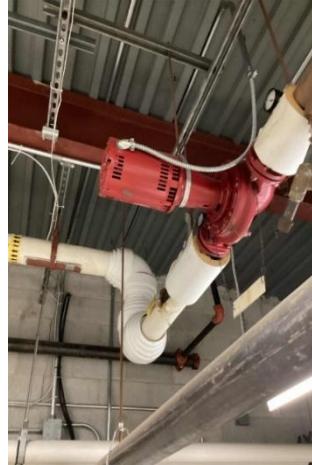
Heating Hot Water Pumps
