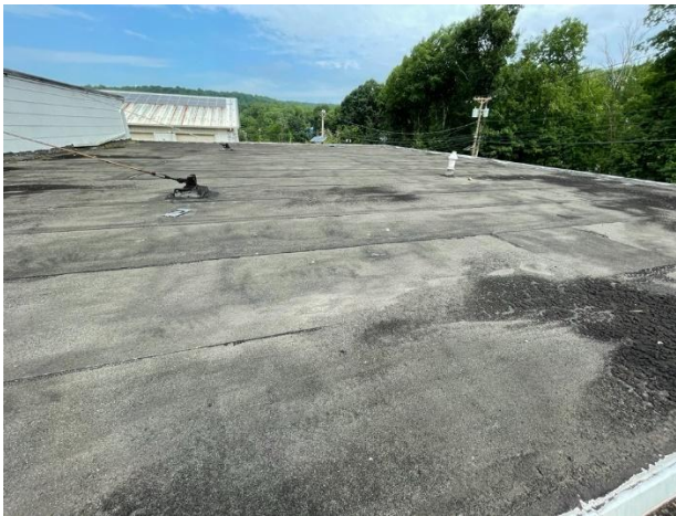
Old DPW Garage Roof
