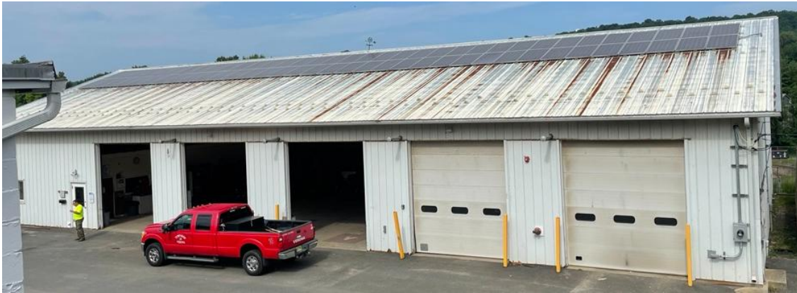
New DPW Garage
