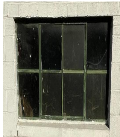
DPW Old Garage Windows
