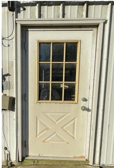
Metal Doors of Garages
