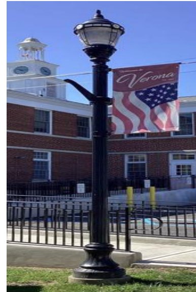
Metal Halide Pole Mount
