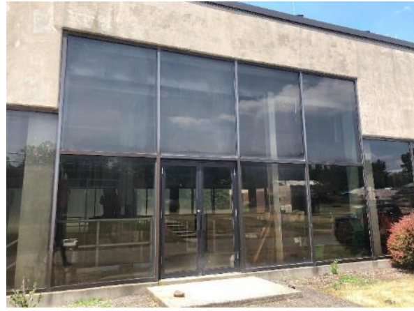
Glass Curtain Wall
