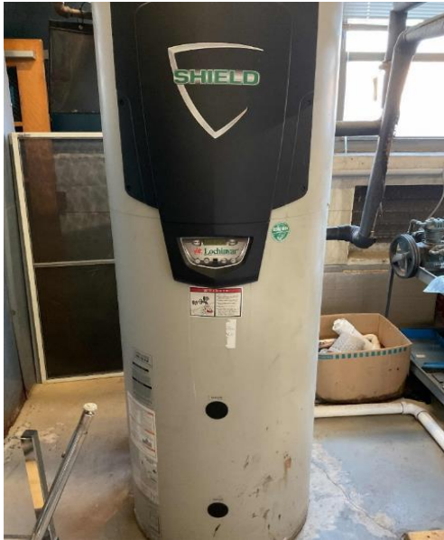
Natural Gas Condensing Storage Tank Water Heater
