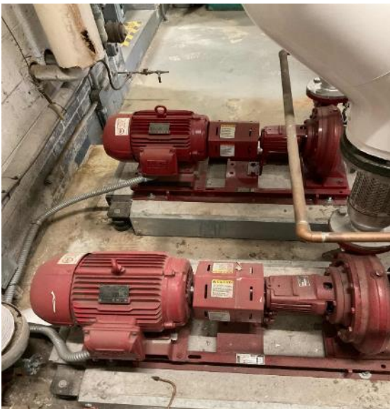
Variable Flow 7.5 Hot Water Pumps
