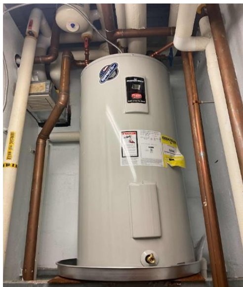
Electric Storage Tank Water Heater
