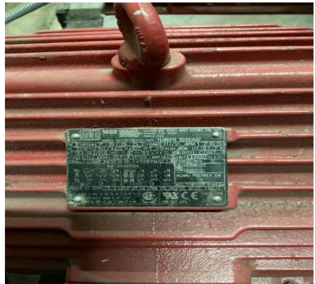
Variable Flow 7.5 Hot Water Pumps
