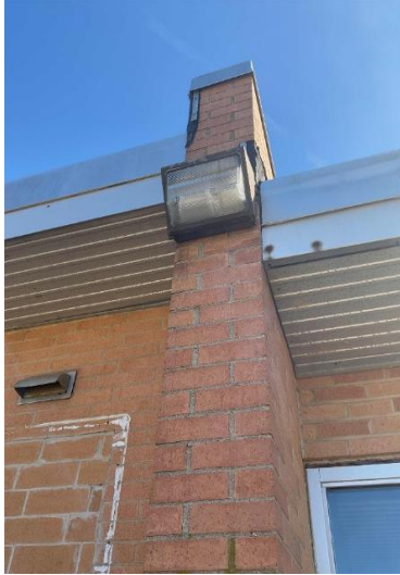
Metal Halide Exterior Wallpacks
