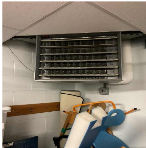
Ceiling Mounted Hydronic Unit Heater
