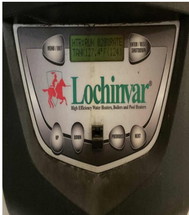
Condensing Gas Fired Storage Tank Water Heater
