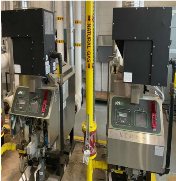
Hot Water Boilers B-1 and B-2
