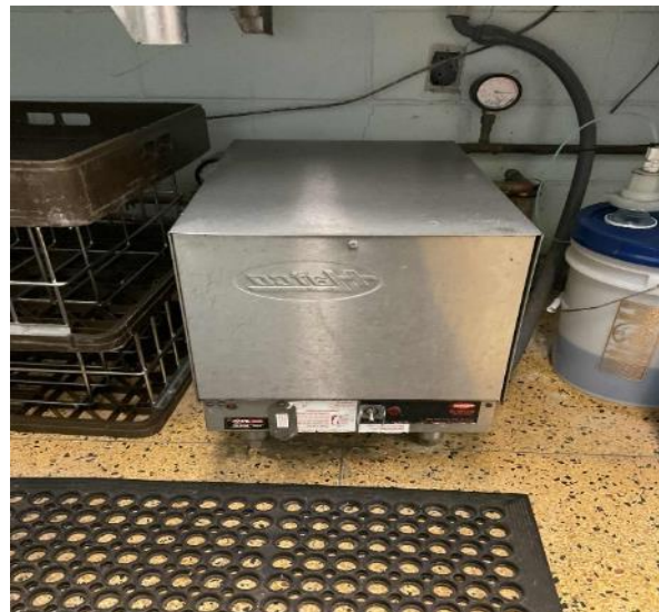
Attached Booster Heater
