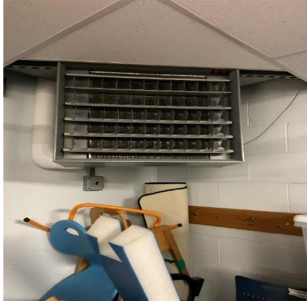
Hydronic Unit Heater
