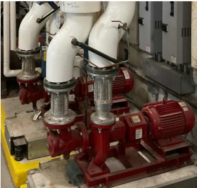
7.5 HP Variable Flow Hot Water Pumps
