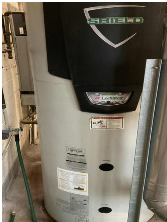
Condensing Gas Fired Storage Tank Water Heater
