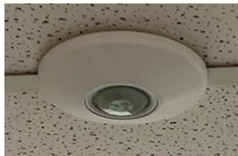
Ceiling Mounted Occupancy Sensor
