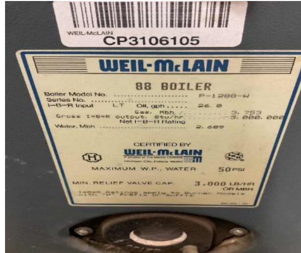
Non-Condensing Heating Hot Water Boilers
