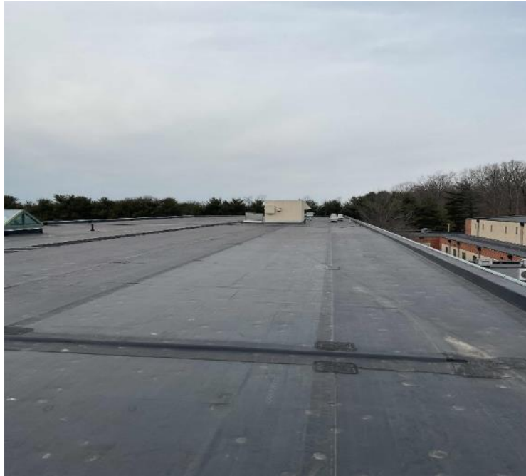
Flat Roof with Black Membrane
