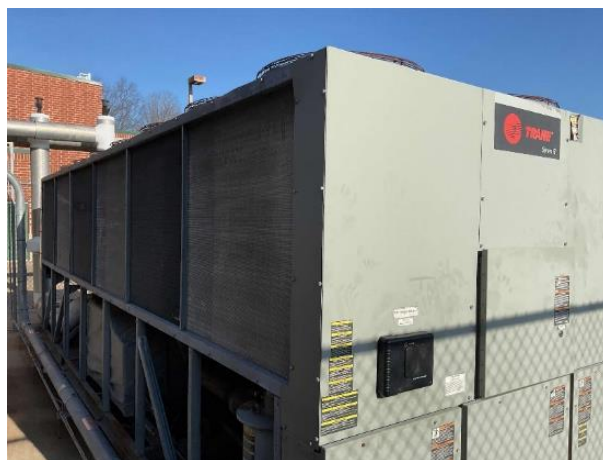
Trane Air-Cooled Screw Chiller
