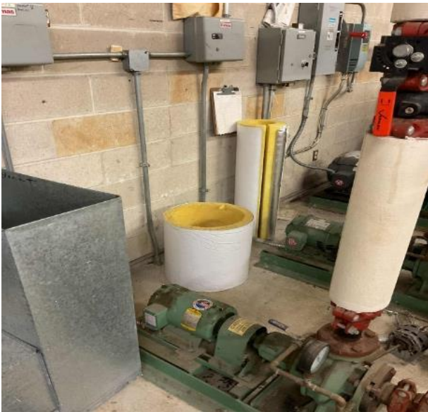
Heating Hot Water Pumps
