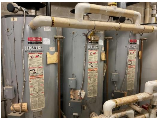
Non-Condensing Storage Tank Water Heaters
