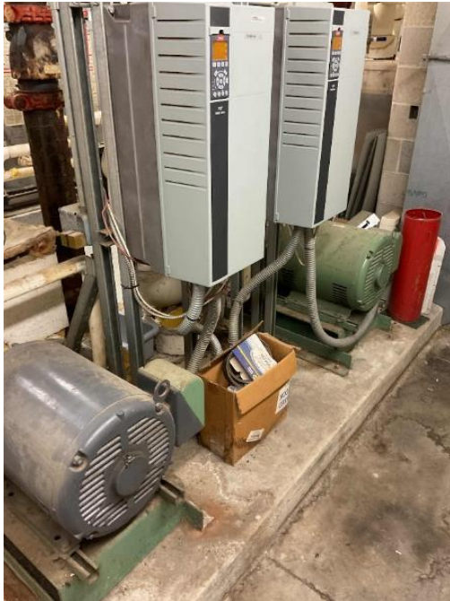
Chilled Water Pumps and Attached VFDs
