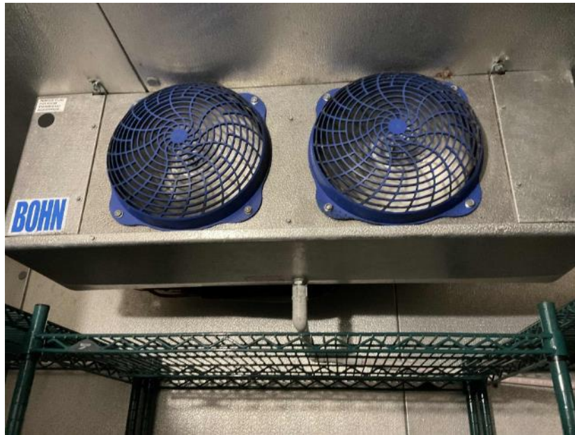
Typical Walk-In Evaporator Unit
