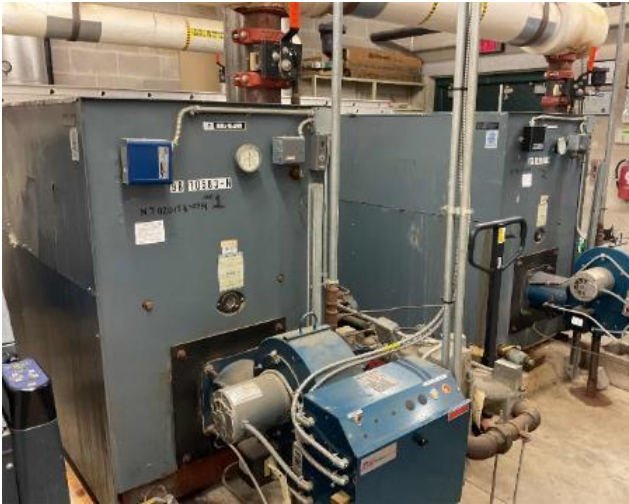
Non-Condensing Heating Hot Water Boilers
