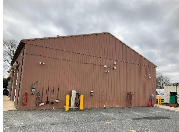
Building Envelope: Exterior Wall Siding
