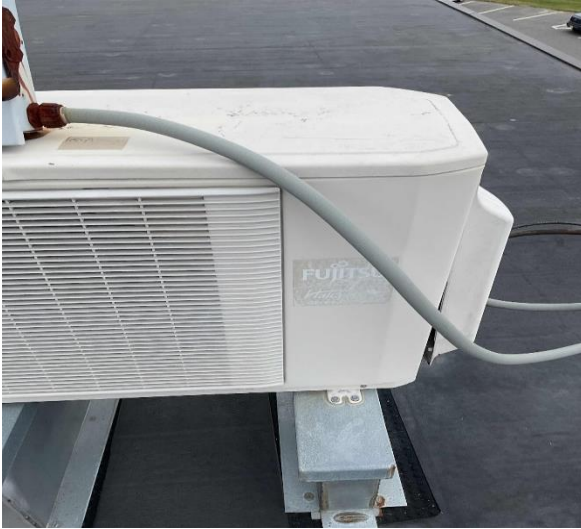
Fujitsu Air-Sourced Heat Pump Outdoor Unit
