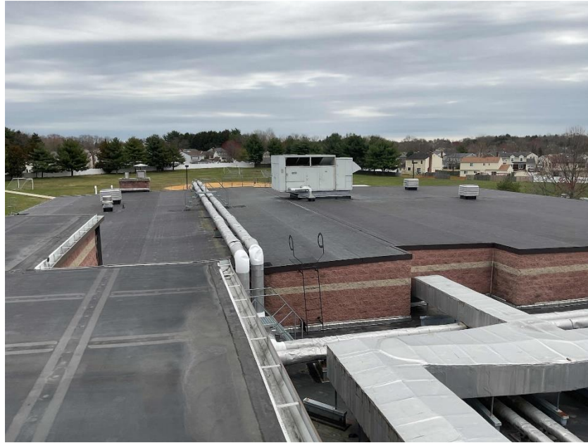
Flat Roof with Black Membrane
