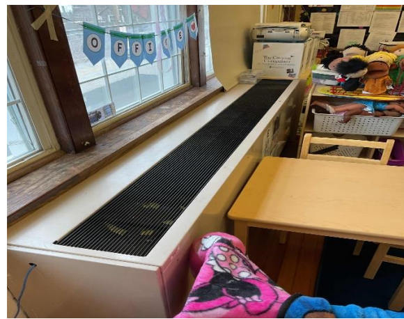
Typical Unit Ventilator in Old Building
