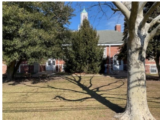
Old Building Exterior Walls
