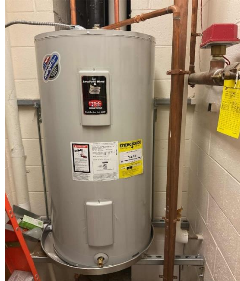
Electric Storage Tank Water Heater in New Building
