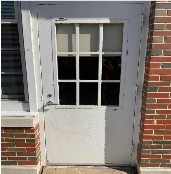
Typical Exterior Doors in New Building
