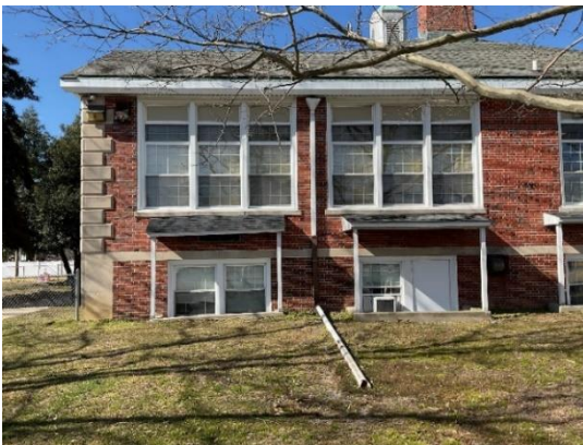
Typical Windows in New Building
