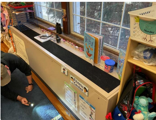
Typical Unit Ventilator in Old Building
