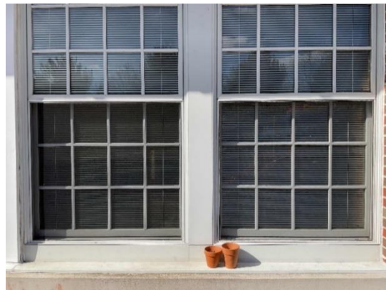
Typical Windows in Old Building
