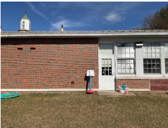
New Building Exterior Walls
