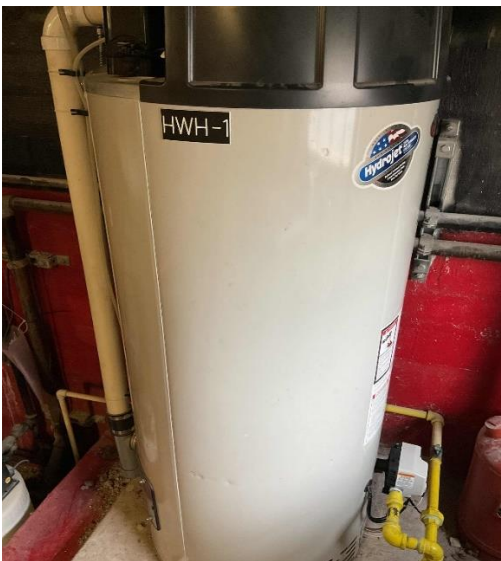
Electric Storage Tank Water Heater in New Building
