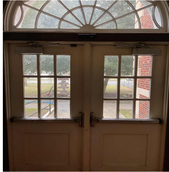
Typical Exterior Doors in Old Building
