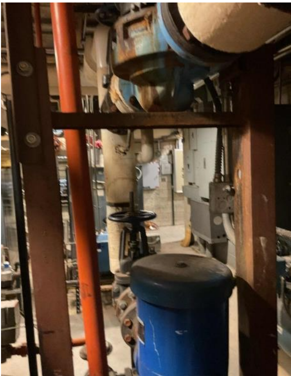
Heating Hot Water Pumps
