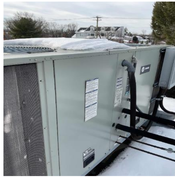
Typical Split-System Air Conditioner Condensing Units on Facility Roof
