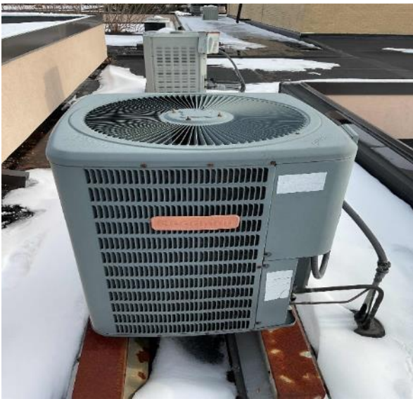
Typical Split-System Air Conditioner Condensing Units on Facility Roof
