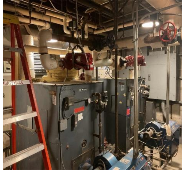
Non-Condensing Boilers
