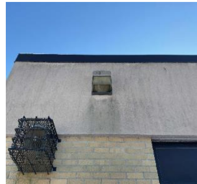
High-Pressure Sodium Exterior Fixture
