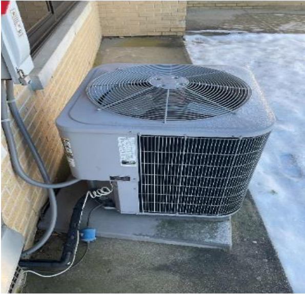
Typical Classroom/Office Condensing Units
