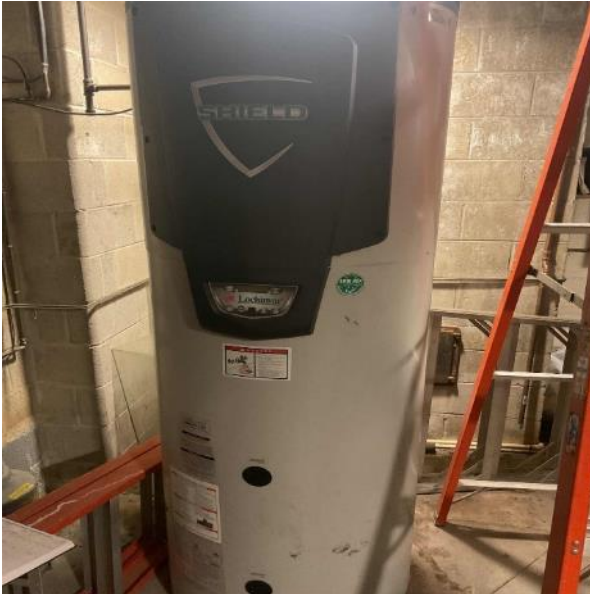
Main Building Natural Gas Hot Water Heater
