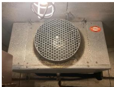
Walk-In Freezer and Cooler Evaporators
