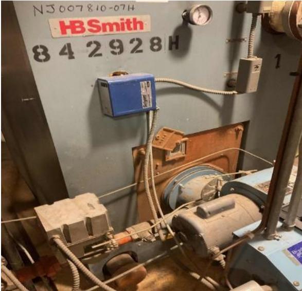
Non-Condensing Boilers
