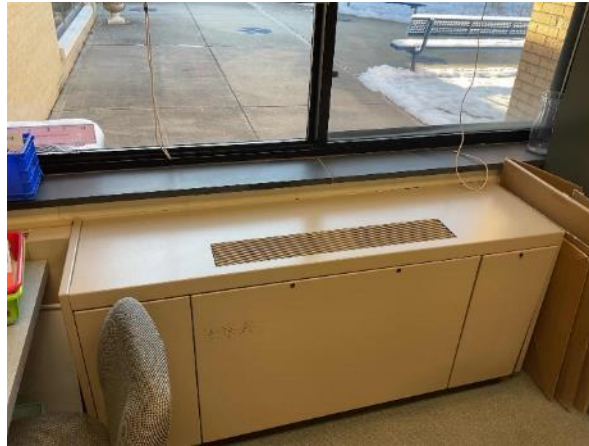
Typical Unit Ventilator
