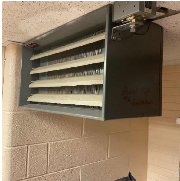
Typical Ceiling-Mounted Hydronic Unit Heater
