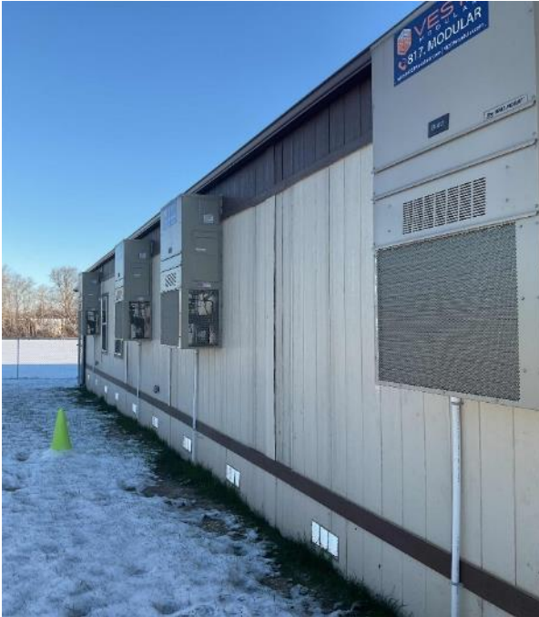
TCU Through-the-Wall Package Air Conditioners
