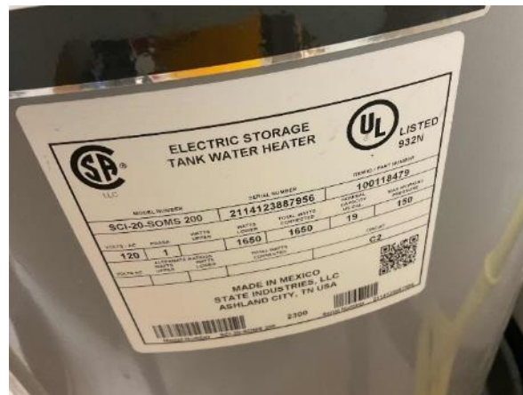
TCU Electric Storage Tank Water Heater
