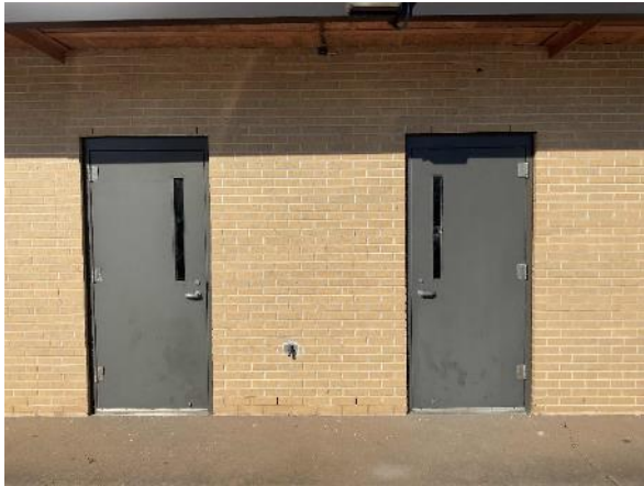
Typical Exterior Doors
