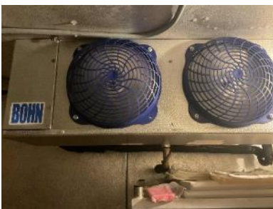
Walk-In Freezer and Cooler Evaporators
