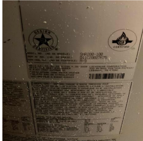
Main Building Natural Gas Hot Water Heater
