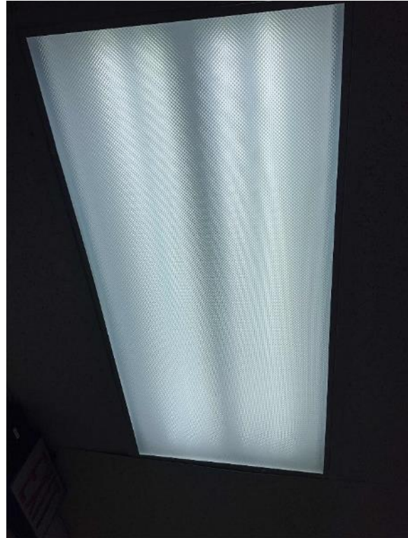
Linear Fluorescent T8 Fixture
