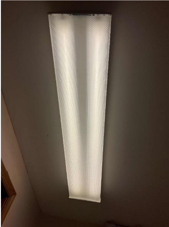
Linear Fluorescent T8 Fixture
