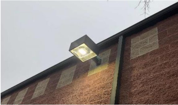
Exterior Pole Mounted LED Fixture
