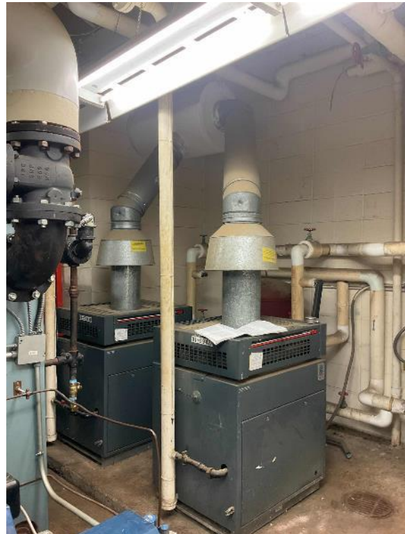
Boiler- Domestic Hot Water Heater
