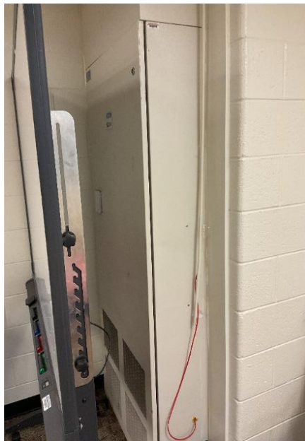
Typical Heat Pump in Classrooms and Offices
