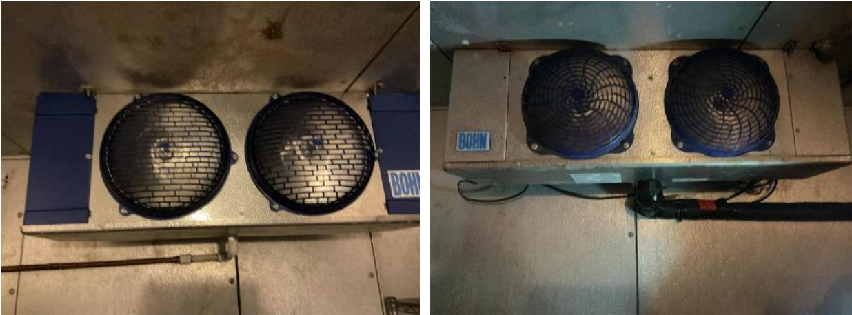
Walk-In Evaporators
