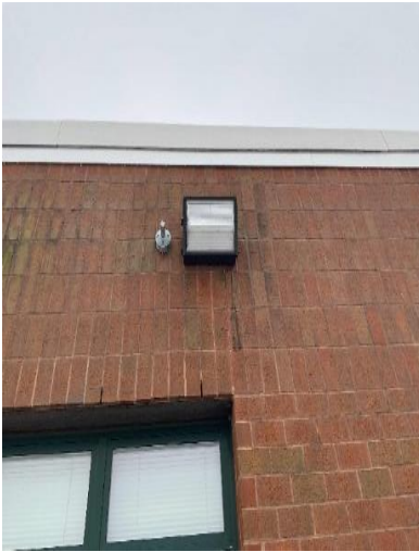
Metal Halide Wall Packs and Lights
