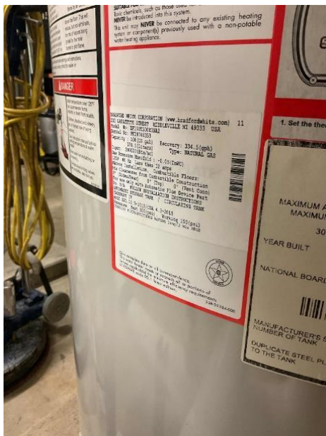
Condensing Natural Gas Water Heater
