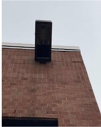
Metal Halide Wall Packs and Lights
