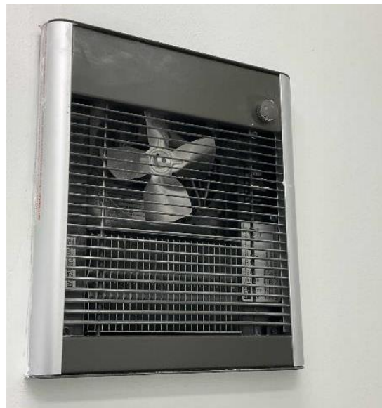
Electric Unit Heater-Pride Pavilion
