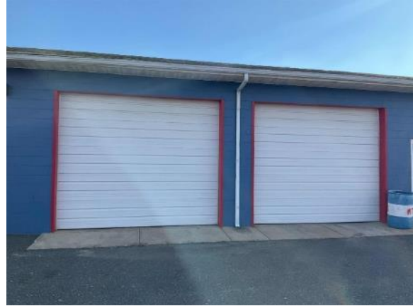
Overhead Doors: O'Brien Hall
